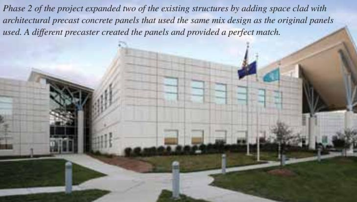
*Phase 2 of the project expanded two of the existing structures by adding space clad with architectural precast concrete panels that used the same mix design as the original panels used. A different precaster created the panels and provided a perfect match.*
