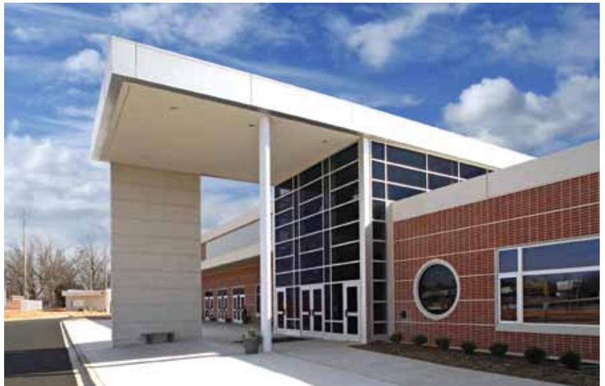
Budget restraints and a search for new delivery methods have brought precast concrete construction to the forefront for many schools. The Carolina High School in Greenville, S.C., was designed by Perkins+Will with a total precast concrete system of load-bearing wall panels and double tees. The project won the award as Best School Design in the 2007 PCI Design Awards competition.
