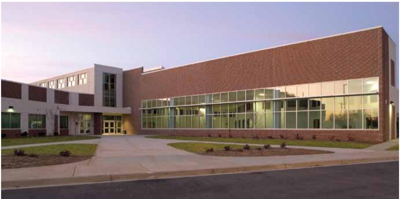
*The new Riverside High School in Greer, S.C., was changed from a major renovation into a project built from scratch after design work showed remodeling costs were exceeding budget. The new school, featuring a total-precast concrete structural system and panels, was built adjacent to the existing school, where class remained underway.*
