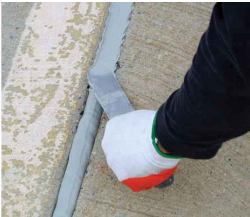
Routine maintenance, such as inspecting and repairing joints, will keep parking structures in good shape and prevent expensive repairs that often result from neglect.
