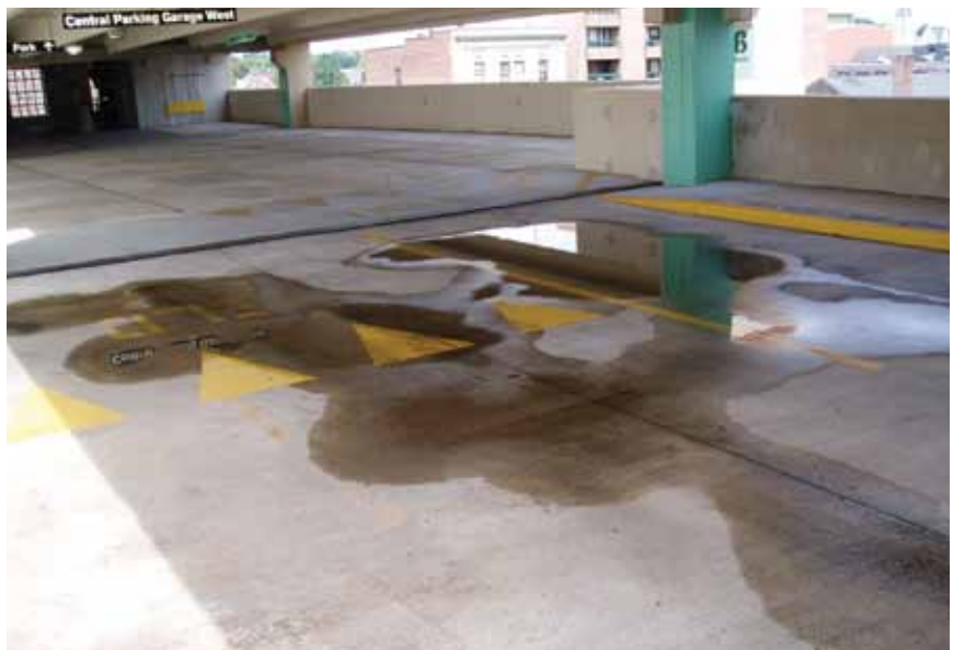
A key goal for designers when planning the structure is to work to eliminate any aspects that encourage water ponding, which can increase water penetration into the concrete and the potential for freeze-thaw damage.
