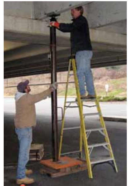
Creating a maintenance program for an existing structure will depend on its age and the amount of maintenance performed over the years. A survey of all conditions should identify immediate safety issues while working to create a three- to five-year plan for restoring the structure's condition.
