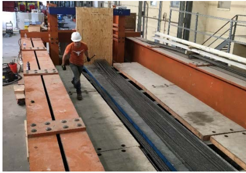
(a) Installing the strands
