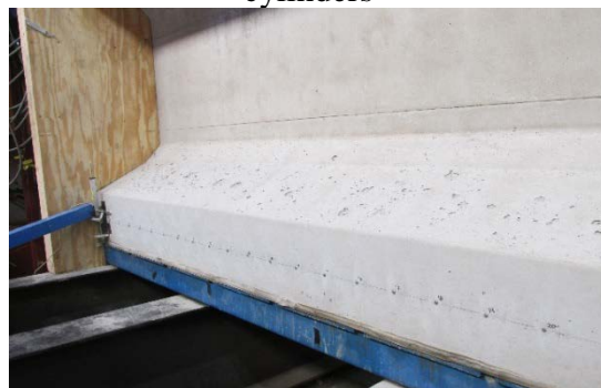
(h) Prestress transfer and inspection
