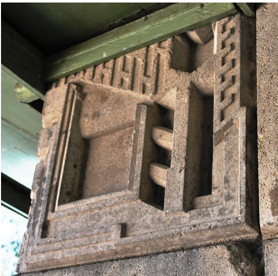
Figs. 10-11 Original dry-cast Freeman block, 1924 A wet-cast Freeman block (McAlister 2009, 123)
