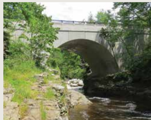
Bottom right photo courtesy of VHB.
