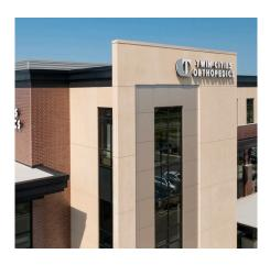
usually follow a consistent exterior facade, the design team tries to do something creative with each new building. This project leveraged precast concrete by replacing the typical metal band seen at the tops of other TCO buildings with more cost-effective prefabricated panels stained to match the metal used in other designs.
