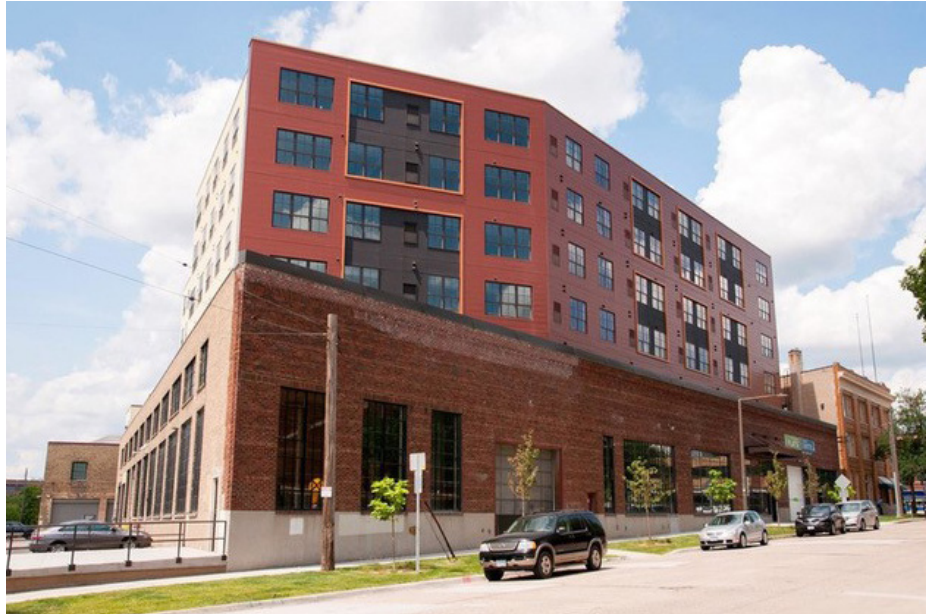
Owner: Steven Scott Management, Inc. • Architect/Engineer: BKV Group • General Contractor: Frana Companies • Hollowcore Erection: Zachman Precast Inc. • Location: St. Paul, MN
