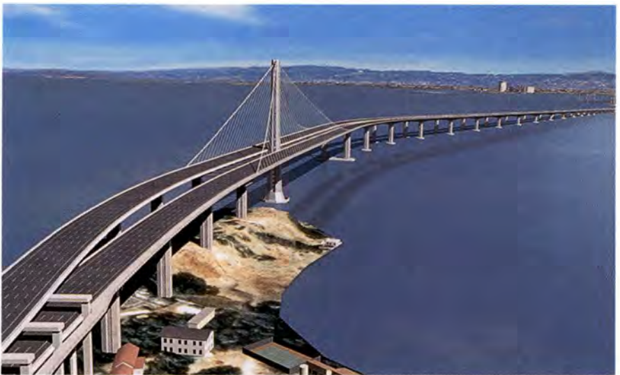
Fig. 25. Proposed cable stayed spans for San Francisco-Oakland Bay Bridge in California.
