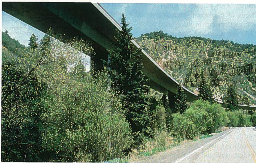
Fig. 1. French Creek Viaduct, Glenwood Canyon, Colorado (precast segmental construction).
