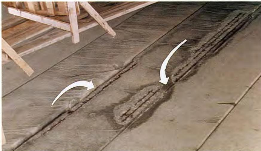
Fig. 4. Corroded prestressed strands on both sides of grouted keyway on bottom side of box beam bridge. Note staining on member.
