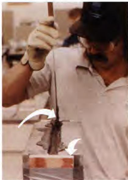
Fig. 9. Consolidation of grout for composite units.
