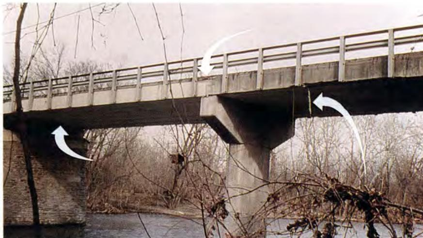
Fig. 5. Midspan replacement of box beam bridge. Arrows show replaced midspan box beams, deck, and hanging broken prestressed tendon from box beam.
