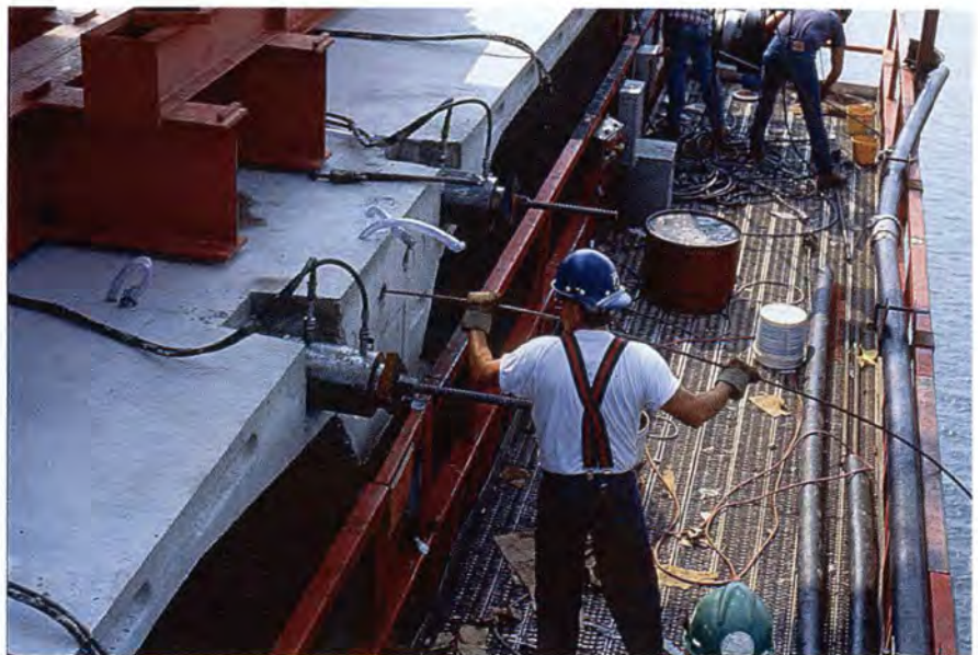
Fig. 22. Cleaning out post-tensioning ducts.
