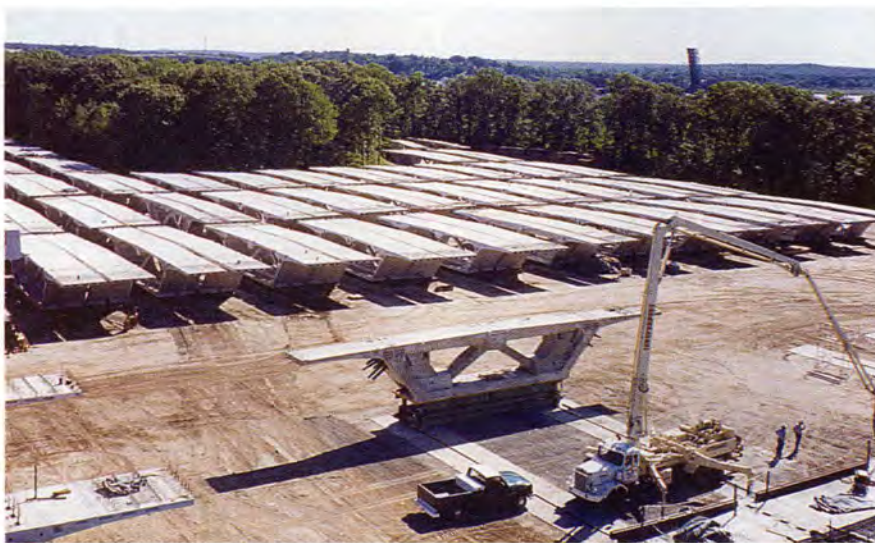
Fig. 7. Segments in storage; total storage capacity of 180 units.
