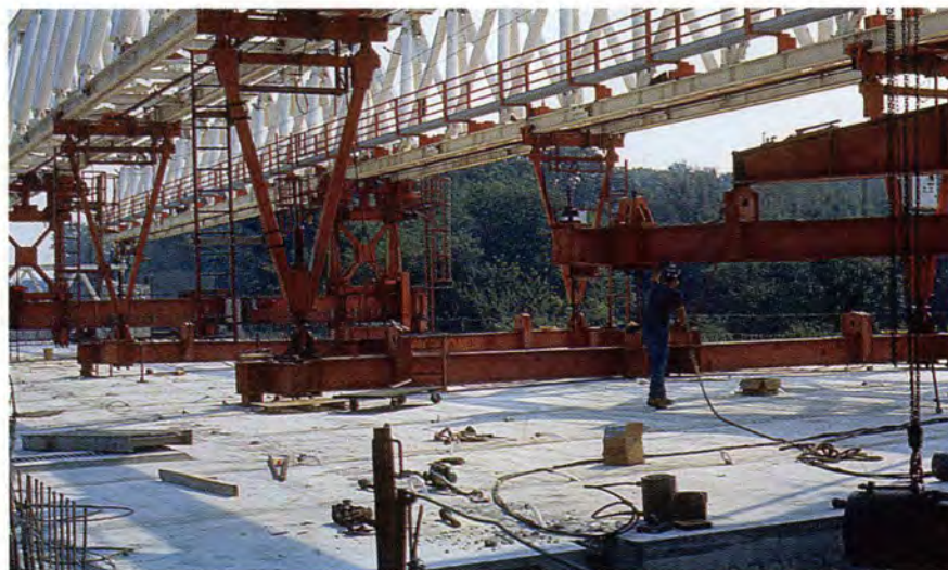
Fig. 26. Gantry stabilizers are connected to the deck.
