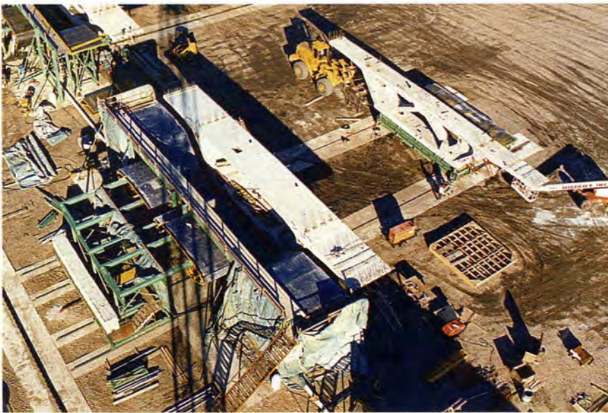
Fig. 6. Short-line match casting of segments.
