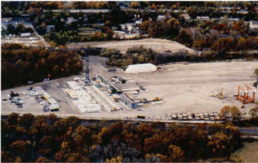
Fig. 5. Casting yard layout.
