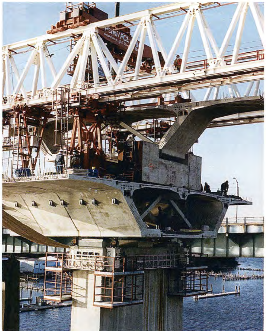
Fig. 23. Pier table complete and segments for cantilevers moving out from pier.
