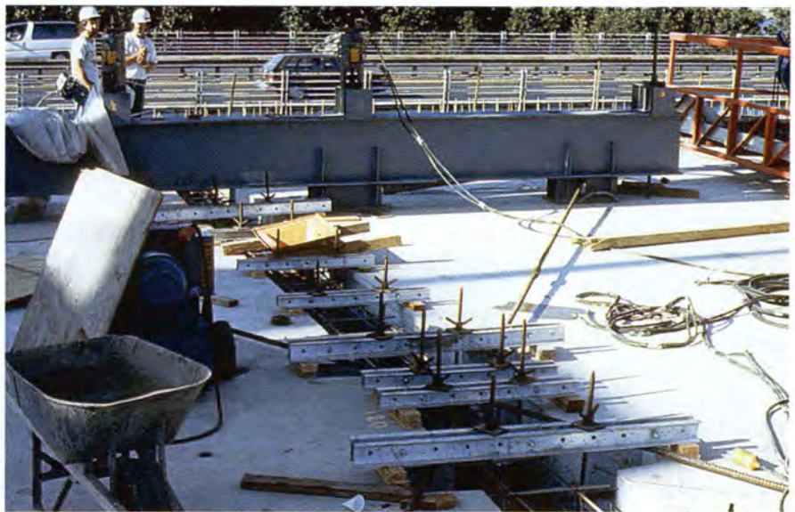
Fig. 27. Final adjustments at the closure gap.
