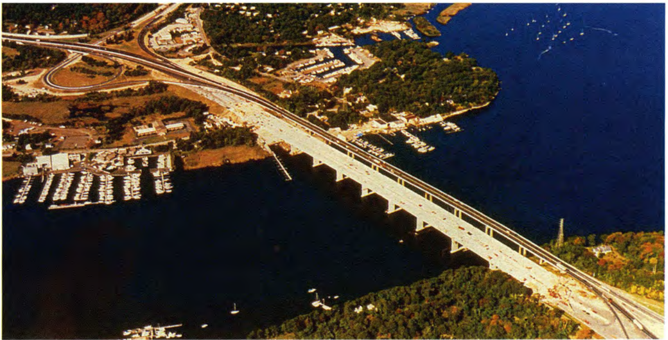
Fig. 1. Overall view of Raymond E. Baldwin Bridge nearing completion.
