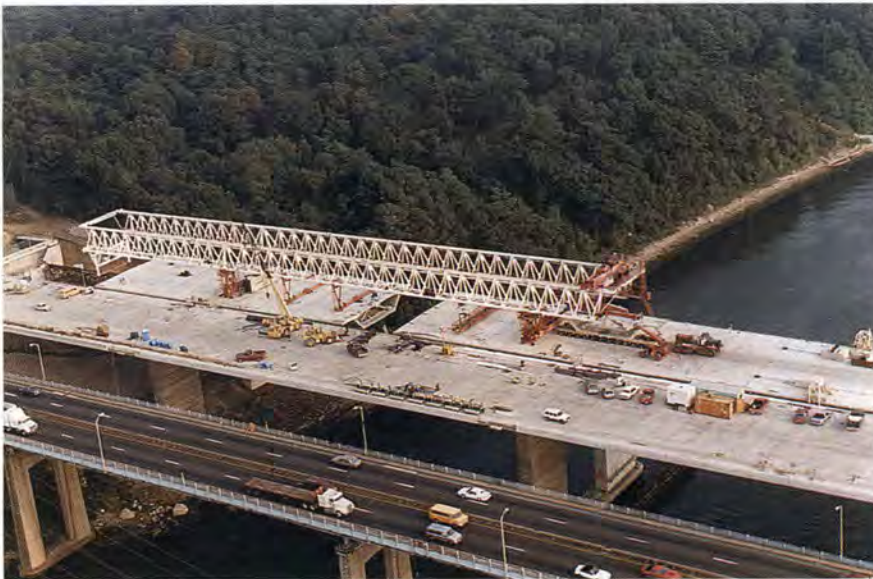
Fig. 15. The 450 ft (137 m) launching gantry.
