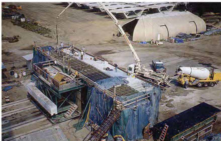
Fig. 12. Concrete placement with a mobile pumping unit; curing blankets provide steam curing enclosure.
