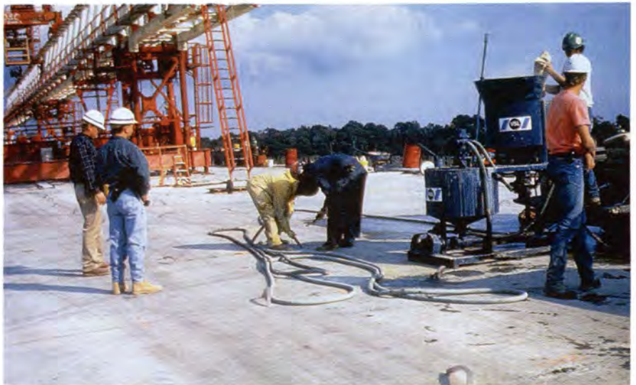
Fig. 28. Grouting operations on a completed span.
