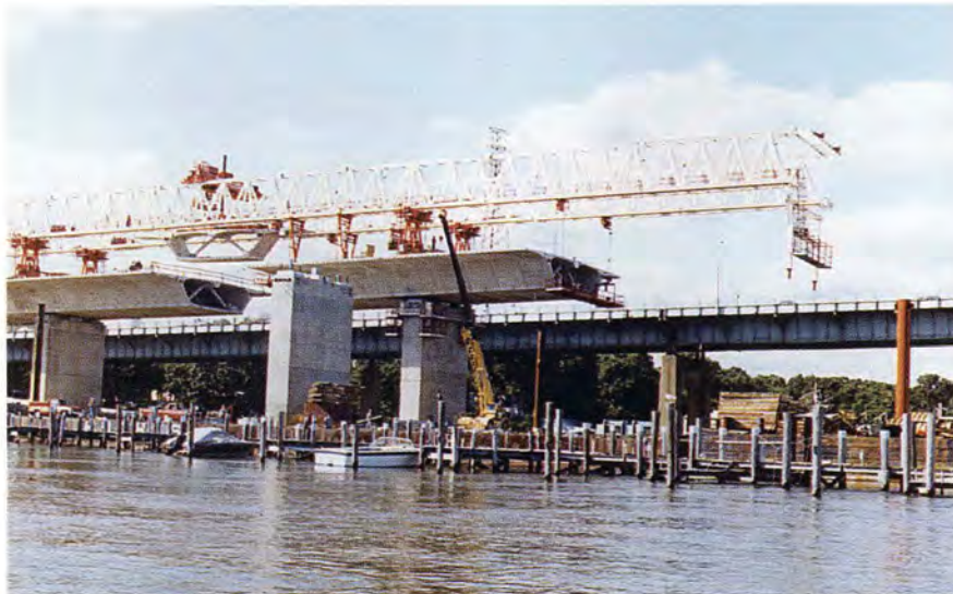
Fig. 25. Cantilever erection by alternately placing segments left and right of the pier.
