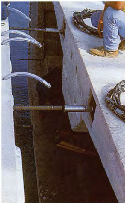
Fig. 19. Connecting the erection post-tensioning bars.
