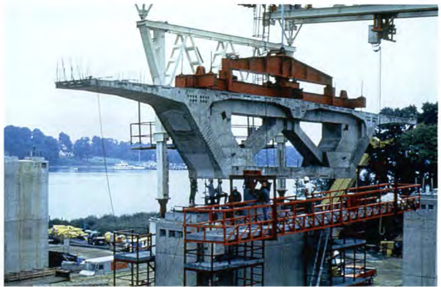
Fig. 17. Pier corbels and pier cap are ready to receive the heavy pier segment.
