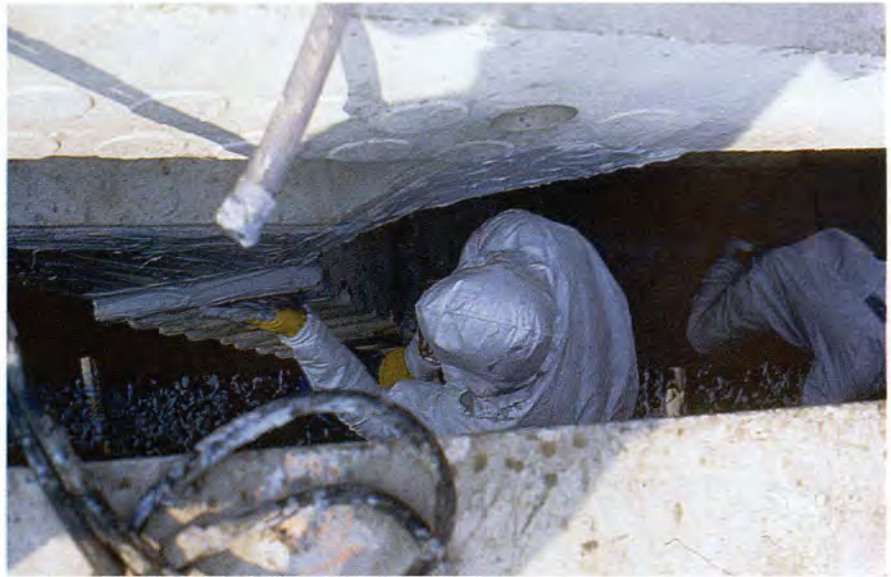
Fig. 20. Applying epoxy adhesive to the joints between segments.
