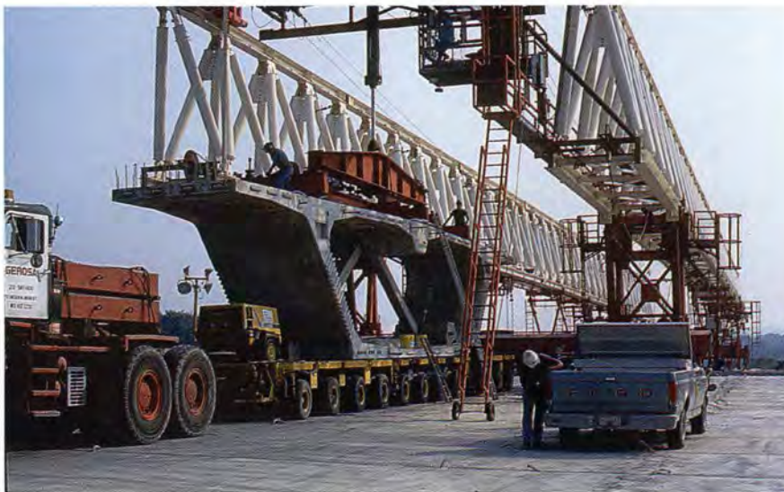
Fig. 16. Segment attached to the gantry lifting beam.
