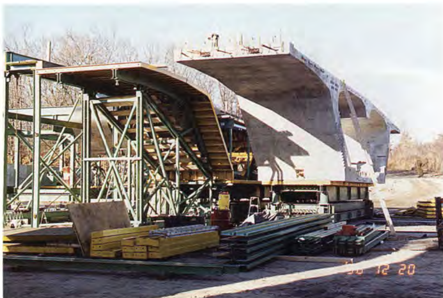
Fig. 11. Setting forms for the match-casting operation.
