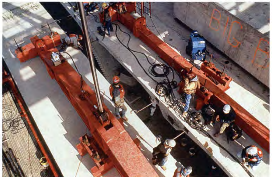
Fig. 18. Second segment at pier.
