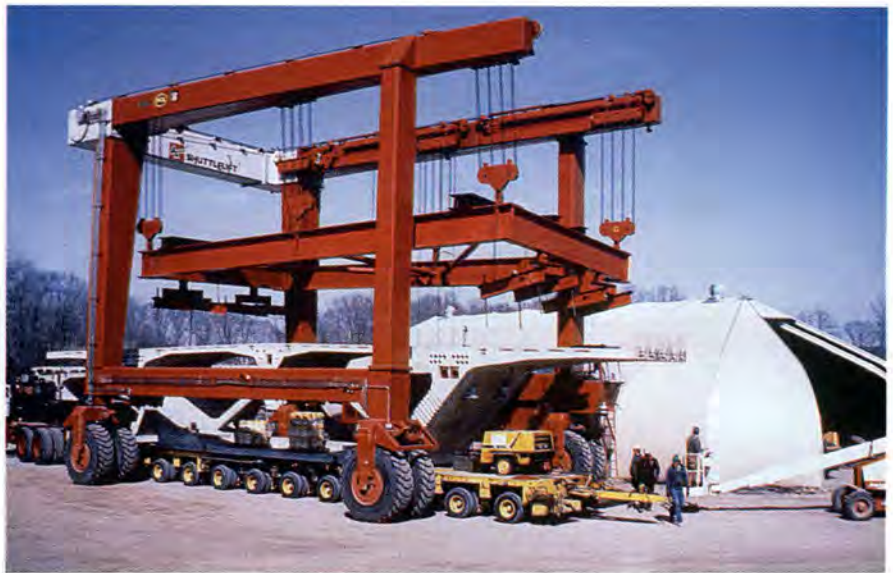
Fig. 13. Precast concrete segment loaded on 96-wheel trailer for transport to site.
