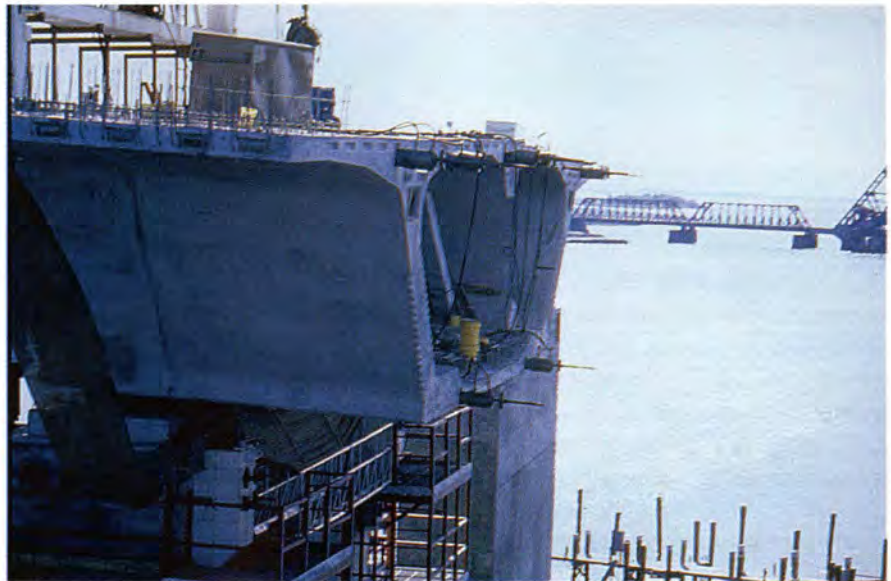
Fig. 21. Second segment post-tensioned to pier segment.
