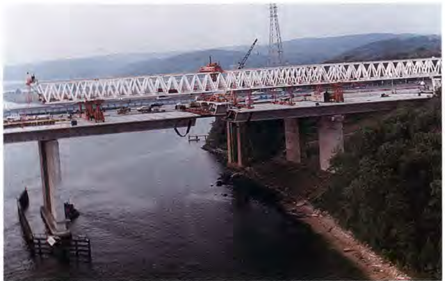
Fig. 30. Raymond E. Baldwin Bridge nearing completion.
