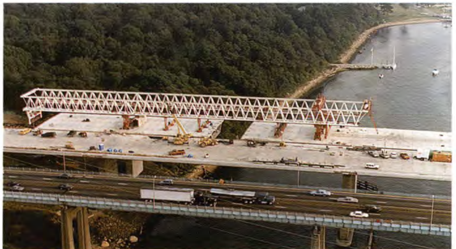
Fig. 29. Final segments being placed in last span of new, parallel segmental bridges; existing bridge is in foreground.
