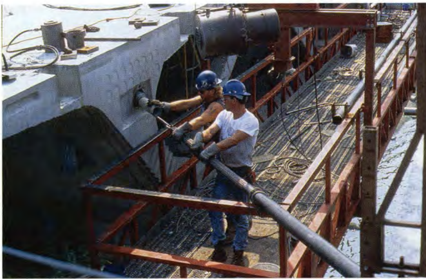
Fig. 24. Inserting permanent post-tensioning tendons into ducts.
