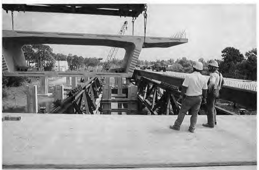
Fig. 14. Segments are lifted by ground based crane onto the erection trusses.
