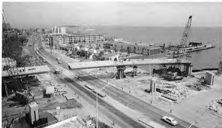
Fig. 12. The first set of cantilevers nears completion across U.S. 90.
