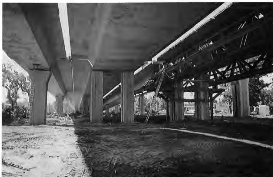
Fig. 16. A series of parallel box girders are later joined together using cast-in-place reinforced concrete closure strips to provide full deck width of ramp transition area.
