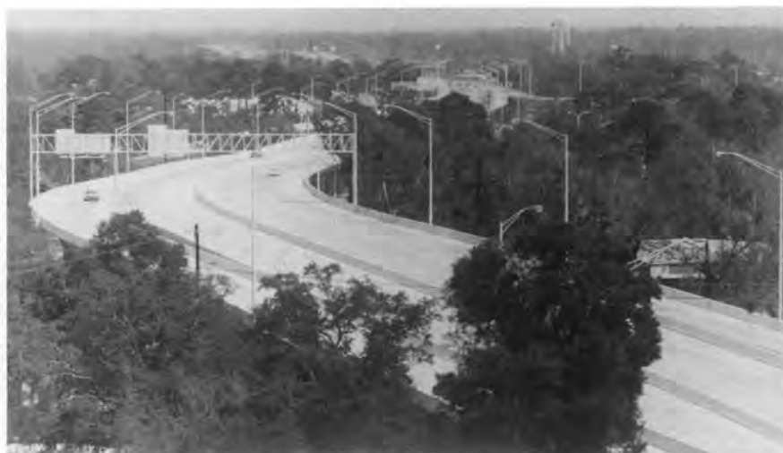
Fig. 2. Aerial view of completed structure with four lanes of traffic and shoulders for a typical width of 81 ft 10 in. (24.9 m).
