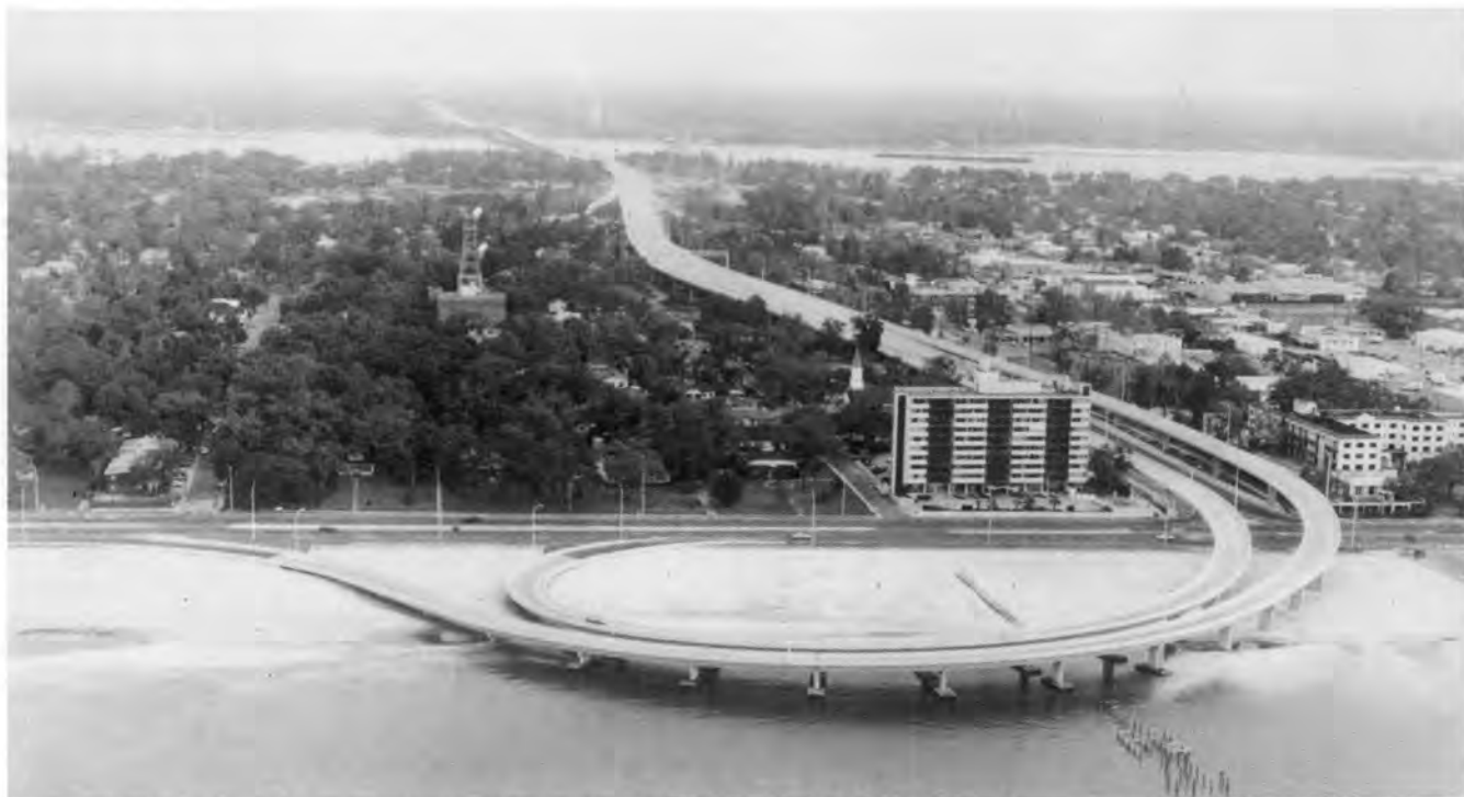
Fig. 1. Panoramic view of Biloxi I-110 viaduct. The 5332 ft (1625 m) mainline urban structure provides four lanes of traffic. Five ramp structures totaling 4830 ft (1472 m) join the mainline facility.
