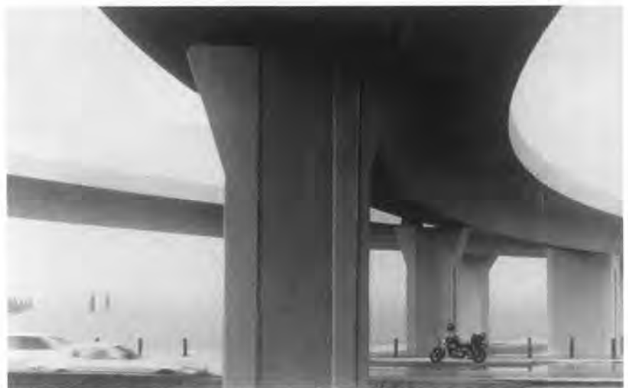
Fig. 19. A view across U.S. 90 of the completed precast prestressed structures. The pier shapes were designed to directly receive the bottom slab of the superstructure in a smooth transition for structural aesthetics.
