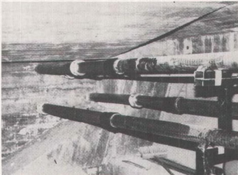
Fig. 19. Reinforced glass fiber duct inside box girder.
