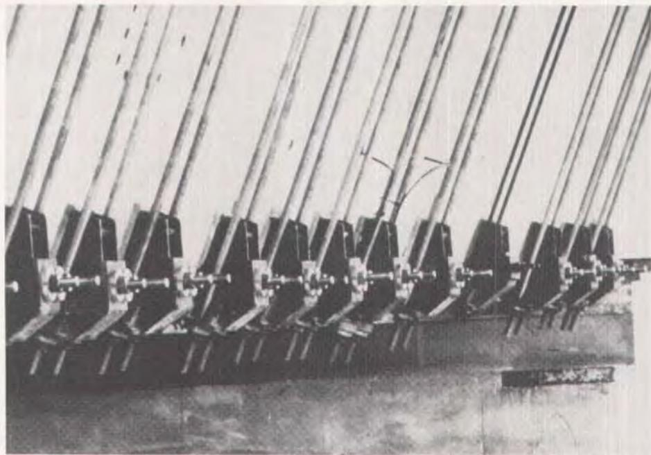
Fig. 15. Steel shoes serving as anchorage for pairs of stainless steel bars.
