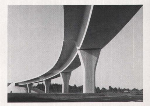
Precast post-tensioned construction provided high quality, plant produced prestressed concrete elements that easily met high strength and exact geometry requirements for this highway interchange bridge in Dade County, Florida.
