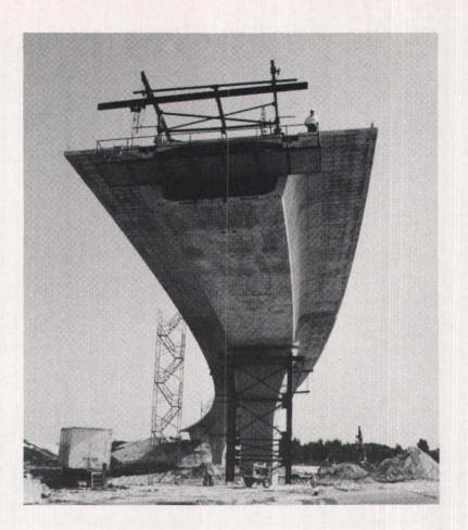
alignment and transfer forces from the superstructure to the foundations. The reinforced concrete piers rest on footings supported on 18 in. (457 mm) square precast prestressed concrete piles of 75 ton capacity.
