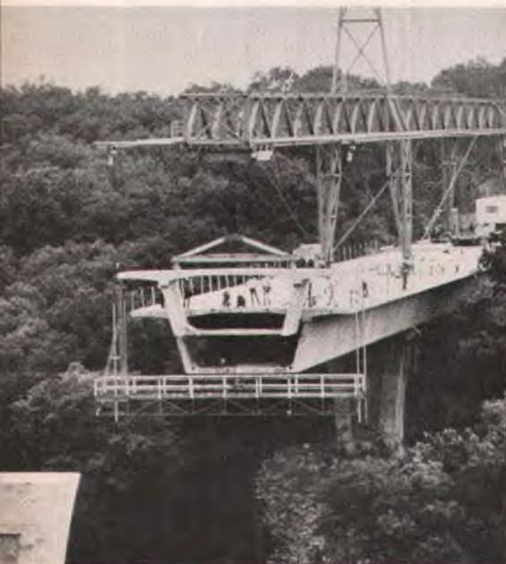
Fig. 3. Launching truss facilitates erection and positioning of bridge segment prior to temporary post-tensioning.
