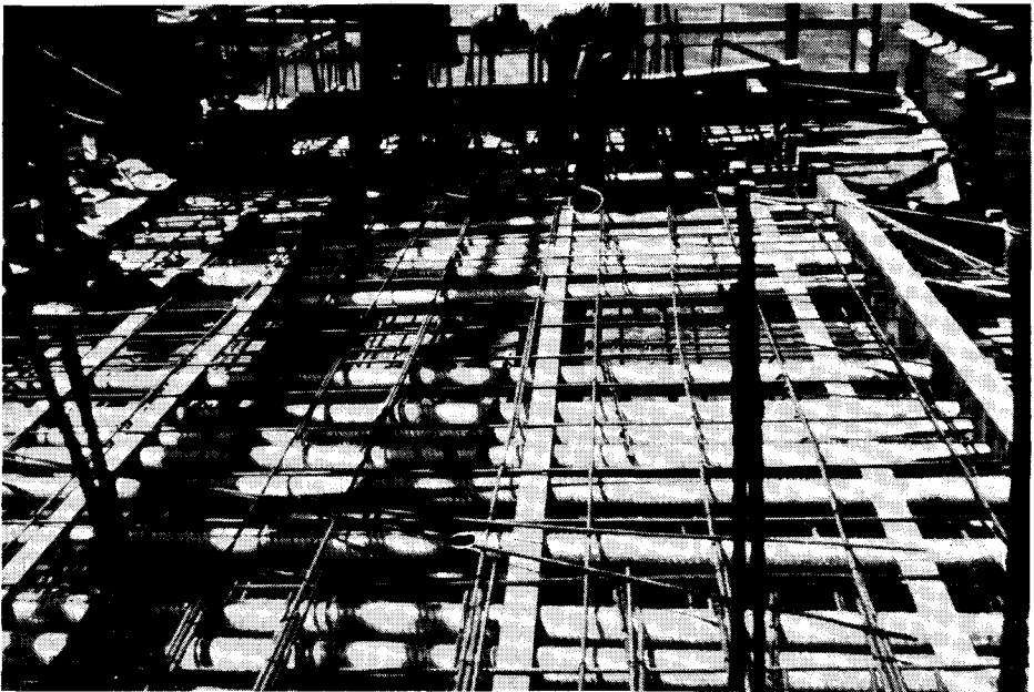
Fig. 15. Tendon installation in the top slab of the Houston Ship Channel Bridge near Houston, Texas.
