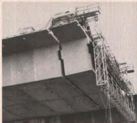
Fig. 13. Segment lifted is ready for application of epoxy to seal the match-cast joint. Note the large single key.
