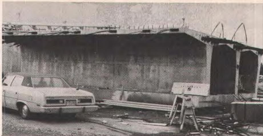
Fig. 8. The 40 x 40 x 8-ft (12.2 x 12.2 x 2.44 m) test section was constructed prior to casting segments.
