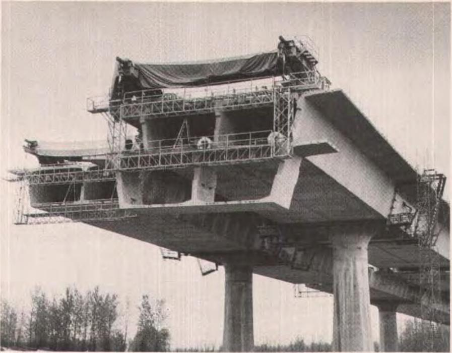
Fig. 24. Precast segment being lifted into place (North Channel section).
