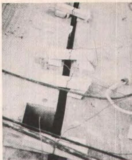
Fig. 19. Ready to place mortar for 2-in. (51 mm) wet joint to adjust alignment and for twist.
