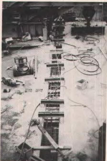
Fig. 12. Ready to make the 1 ft 9 in. (0.534 m) closure pour between the first segment and the pier table.
