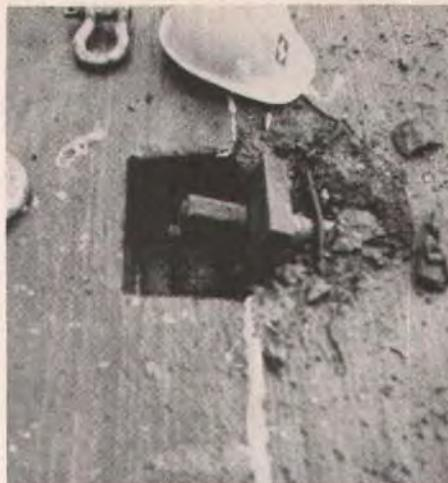
Fig. 15. Crushing of concrete behind the bearing plate of one of twelve temporary stress rods used to apply compression to match-cast joints. Rods are removed when permanent tendons have been stressed.
