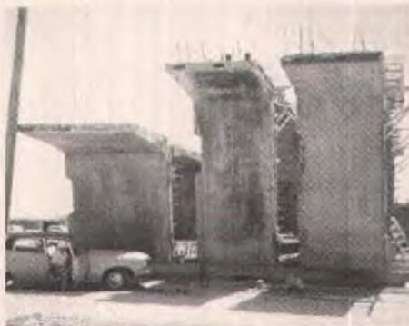
Fig. 10. 12 and 17-ft (3.66 and 5.18 m) deep segments shown in storage. All three precast segments shown are elements which will be adjacent to pier tables.
