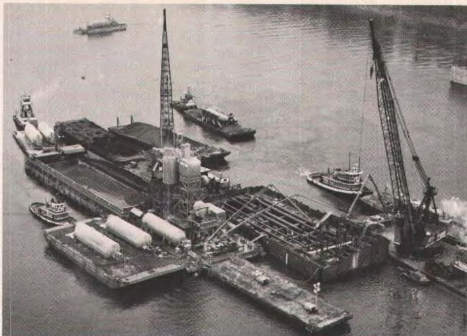
Fig. 5. Placing concrete by the tremie method for the 50 x 150 x 39-ft (15.2 x 45.7 x 11.9 m) deep seal at Pier 13. Placement of the concrete for the seal was completed in 55 hours.
