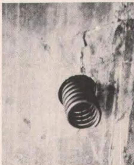
Fig. 16. To develop additional load transfer at a match-cast joint in which the epoxy did not set, 4-in. (102 mm) diameter holes were cored into the joint and filled with spiral reinforced high strength mortar.
