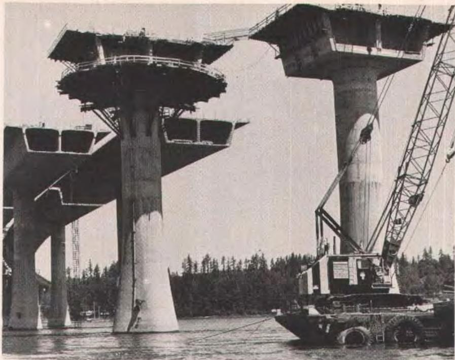
Fig. 26. Construction progress showing the cast-in-place pier tables and the advancing precast prestressed superstructure (North Channel section).
