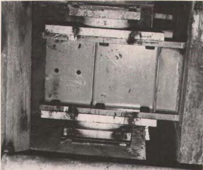
Fig. 22. Hinges with opposing pot bearings at midspan.
