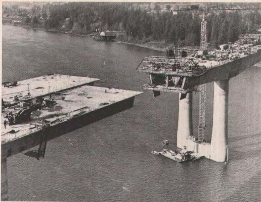
Fig. 30. The 176-ft (54 m) cantilevers on left (foreground) are made up of precast segments. On the right is the cast-in-place segmental cantilever from Pier 13.
