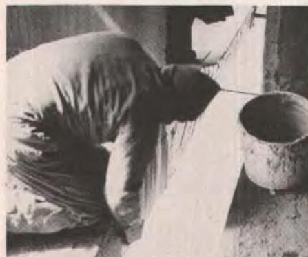
Fig. 14. Application of epoxy to match-cast face.
