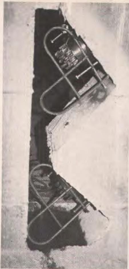
Fig. 17. Blockouts in the adjacent segments opposite the draped tendon anchorage, when filled with concrete, provided additional shear keys.
