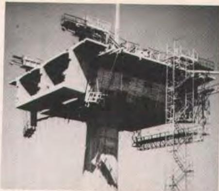
Fig. 11. Lifting the first segment with closure forms attached.
