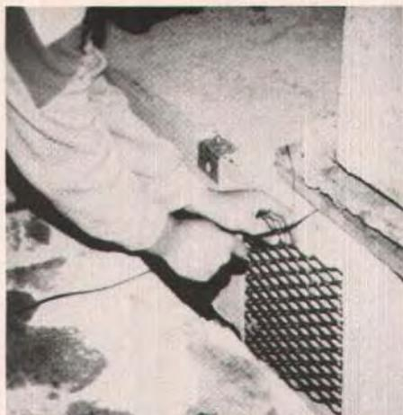
Fig. 18. Expanded metal shims  $\frac{1}{8}$  in. (3.2 mm) thick being placed in joint in attempt to adjust alignment. In shimming a joint, approximately 1000 sq in. (0.645 m<sup>2</sup>) of shims were placed in the top or bottom slab at the webs.
