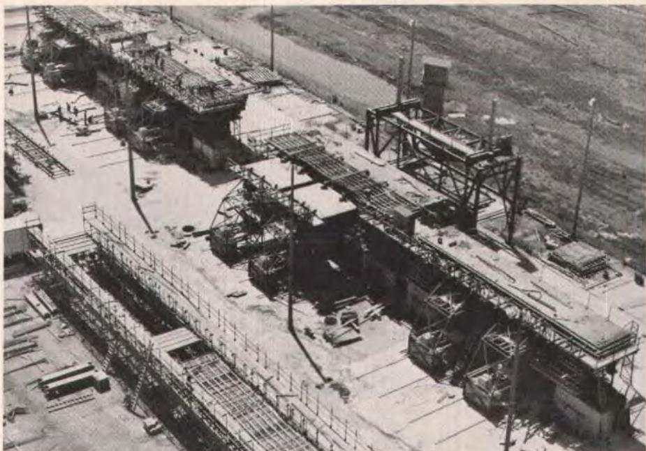
Fig. 9. Four casting machines were used in manufacture of precast segments. Tower in background is for survey control. In foreground are the reinforcing steel templates.
