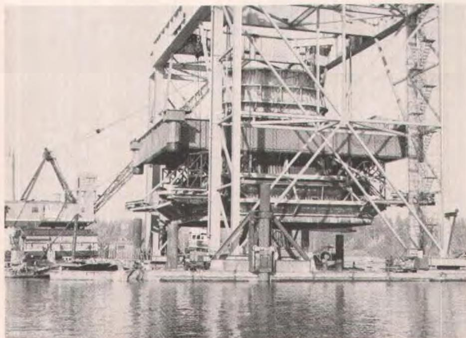
Fig. 4. Preparing to lower the 58 x 76 x 63-ft (17.7 x 23.2 x 19.2 m) high-welded bell-shaped steel form.
