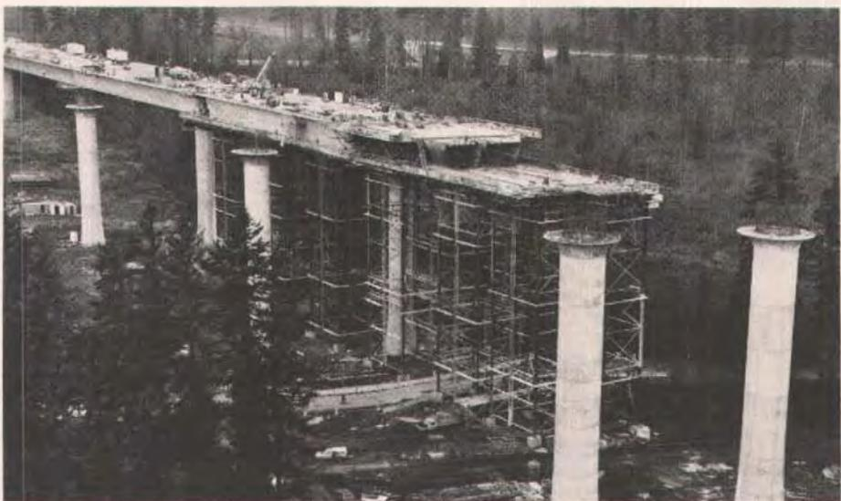
Fig. 6. The Washington Approach spans were constructed by pouring concrete in-place for 71-ft (21.7 m) segments. Falsework up to 120 ft (36.6 m) high supported the spans.
