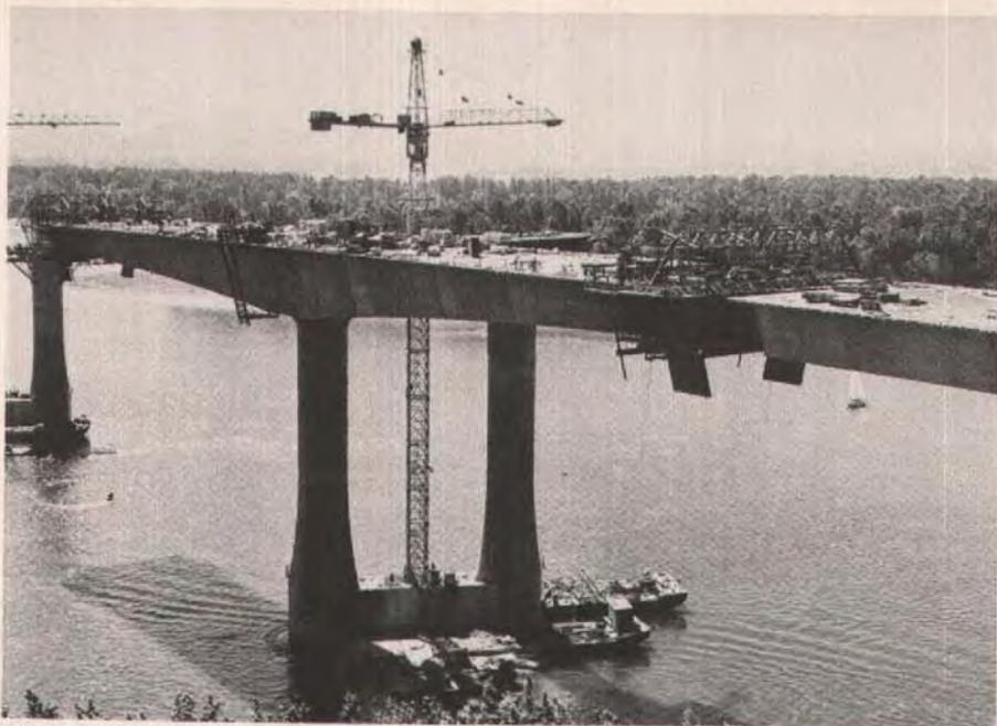
Fig. 28. Nearing completion of the 480-ft (146 m) Span 11 adjacent to the main 600-ft (183 m) span.
