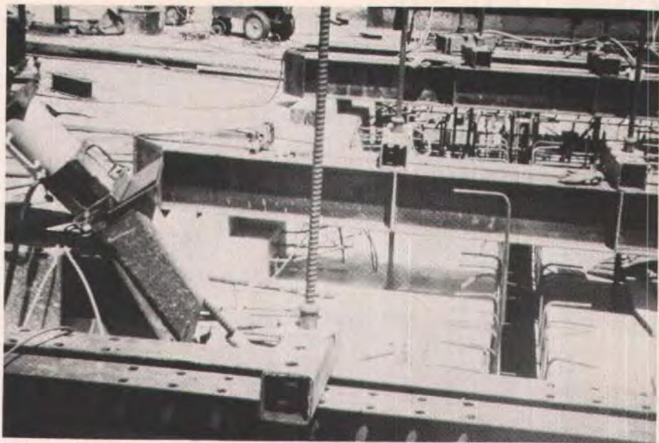
Fig. 21. Forms in place for closure pour. The diagonal stress rod in the bottom left of the picture was used for alignment adjustment and maintaining alignment during the closure pour.
