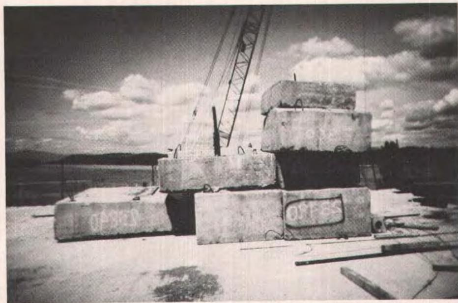
Fig. 20. Weight to produce an unbalancing load of up to 100 kips (445 kN) was placed on the end of the cantilever to adjust alignment.
