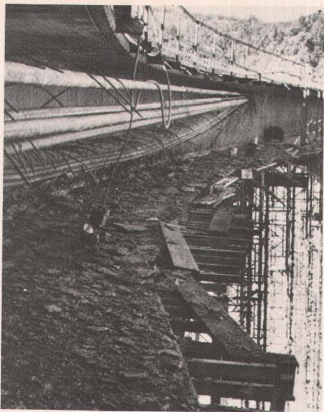
Fig. 5. Curved tendons forcing themselves out of the webs of a segmental box (Las Lomas Bridge, California).
