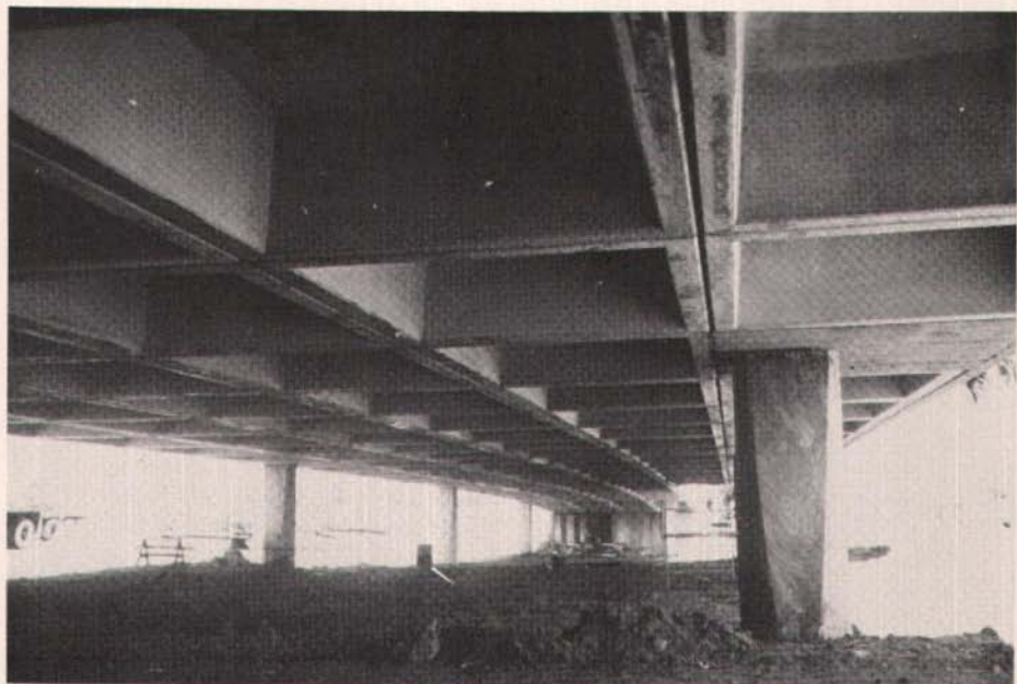
Fig. 9. Airport Bridge, San Juan, Puerto Rico. Constructed with waffle segments.
