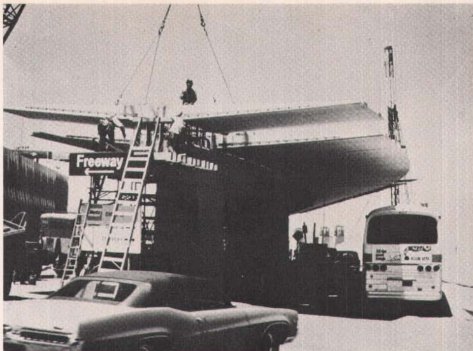
Fig. 10a. San Francisco Airport Elevated Roadway Bridge. Built of precast wing segments without match casting or epoxy joinery.
