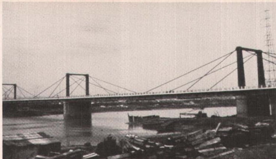
Fig. 7. Kwang Fu Bridge, Taiwan. Constructed with I-girders placed along four panels at 125 ft (38.1 m) forming a 500-ft (153 m) cable-stayed segmental bridge.
