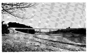
The best looking bridge on such slender single columns was designed by Finsterwalder for the Elztal viaduct, with spans of about 120 ft. The shallow slab is thickened by a flat, mushroom cap to get the necessary fixity with the columns, which are as high as 320 ft.! Many examples already prove that continuous beams on rather high, slender piers least disturb the beauty of the landscape.
