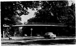
The above pedestrian bridge is a very slender, hollow-plate structure resting on two columns, strengthened at the top by means of a flat cone. Again, a rather deep fascia beam and different colors increase the appearance of slenderness. The structure ends at rather low points in order to reduce the size of the abutments.
