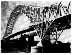
A second example of lack of order and of good proportions is this highway bridge with a span of about 1000 ft. The lattice work of this large arch, and especially the lateral bracing, do not show good order.
