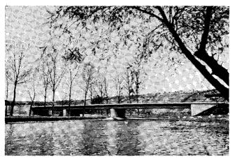
For multi-span river bridges with straight grade, it is preferable to have beams with parallel edges on heavy piers and abutments with parallel wing walls.
