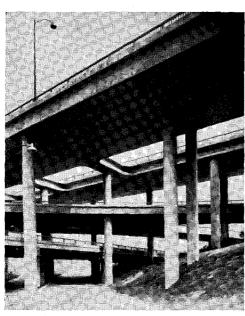
An excellent example of obtaining good order, by reducing the number of structural elements to a minimum, is the first four-level crossing in the world near Los Angeles. This difficult design was solved with two elements only—solid slabs and circular columns. This structure has high aesthetical value.
