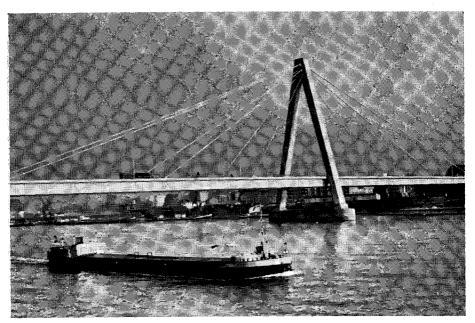
During the last 15 years, bridges have been developed in Germany with different types of stay cables, suspending continuous beams, So far mostly steel bridges have been built, like this bridge crossing the Rhine in Cologne.
