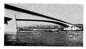
For multi-span bridges with parallel edges, single columns with a cap also give good appearance. The cap, however, must be limited to good proportions in relation to the width of the structure. Caps look bad if they are as wide or even wider than the hollow-box beam.
