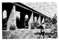
In the design of valley bridges, the development was from heavy and wide masonry piers to slender columns. An old bridge on the Autobahn shows masonry piers fitting well into the free landscape, but almost closing the view into the valley.
