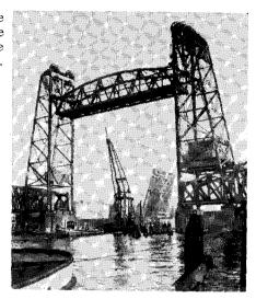
Trusses can be designed to give a good appearance if the chords are parallel and if the diagonal bars have only two directions, as this steel truss bridge may show. In addition to order of directions, there must be good proportions between the chord members and diagonal bars.
