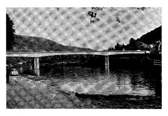
bottom and top lines are parallel or almost parallel. Further, there should be a good proportion between the visible depths at the pier and at mid-span. If the depth is changing too much, then the impression is less favorable. Similarly, the bottom and top edges should be parallel for some length at the ends of the side spans, especially if the bridge is joined to further spans.
