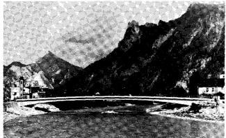
One of the best looking river crossings is this single-span beam bridge, encastered at both ends, over the River Traun in Austria. It is the slenderness and graceful curvature of all lines which makes it so attractive.
