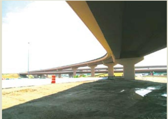
**Figure 4.** Summit Engineering Group designed a U-shaped, precast, post-tensioned concrete box-girder bridge for Interstate 270 that spans Interstate 25 just north of the U.S. Route 36 and Interstate 76 interchange in Denver, Colo. Courtesy of Gregg Reese, Summit Engineering.
