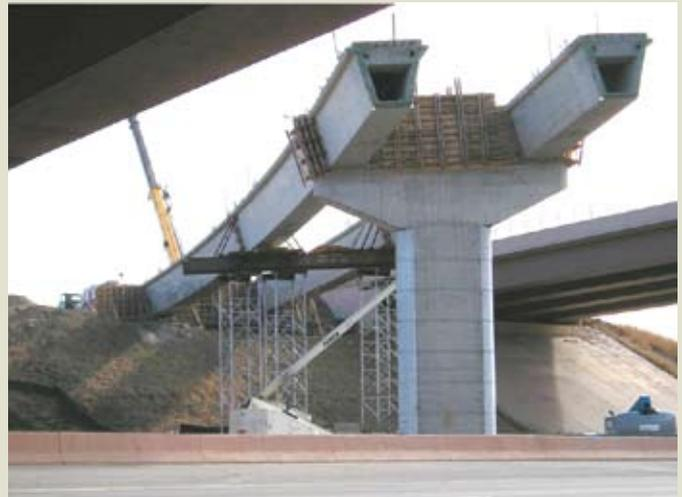
**Figure 5.** The 100-ft-long segments were cantilevered from the piers and supported by temporary shoring for the Interstate 270 bridge in Denver, Colo. Note: 1 ft = 0.305 m. Courtesy of Gregg Reese, Summit Engineering.
