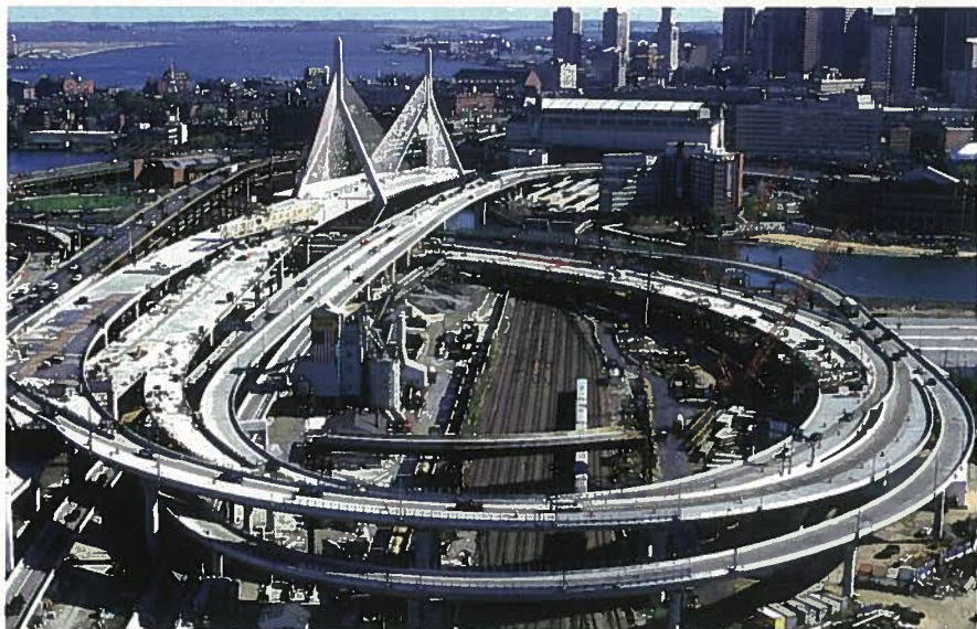
Fig. 14. An aerial view of the I-93 ramps illustrates traffic congestion all-to-familiar to Boston, Massachusetts, commuters. Horizontal curvature as small as 212 ft (64.6 m) and other precast concrete design advantages saved the Massachusetts Turnpike Authority over $27 million at the time of bidding.
