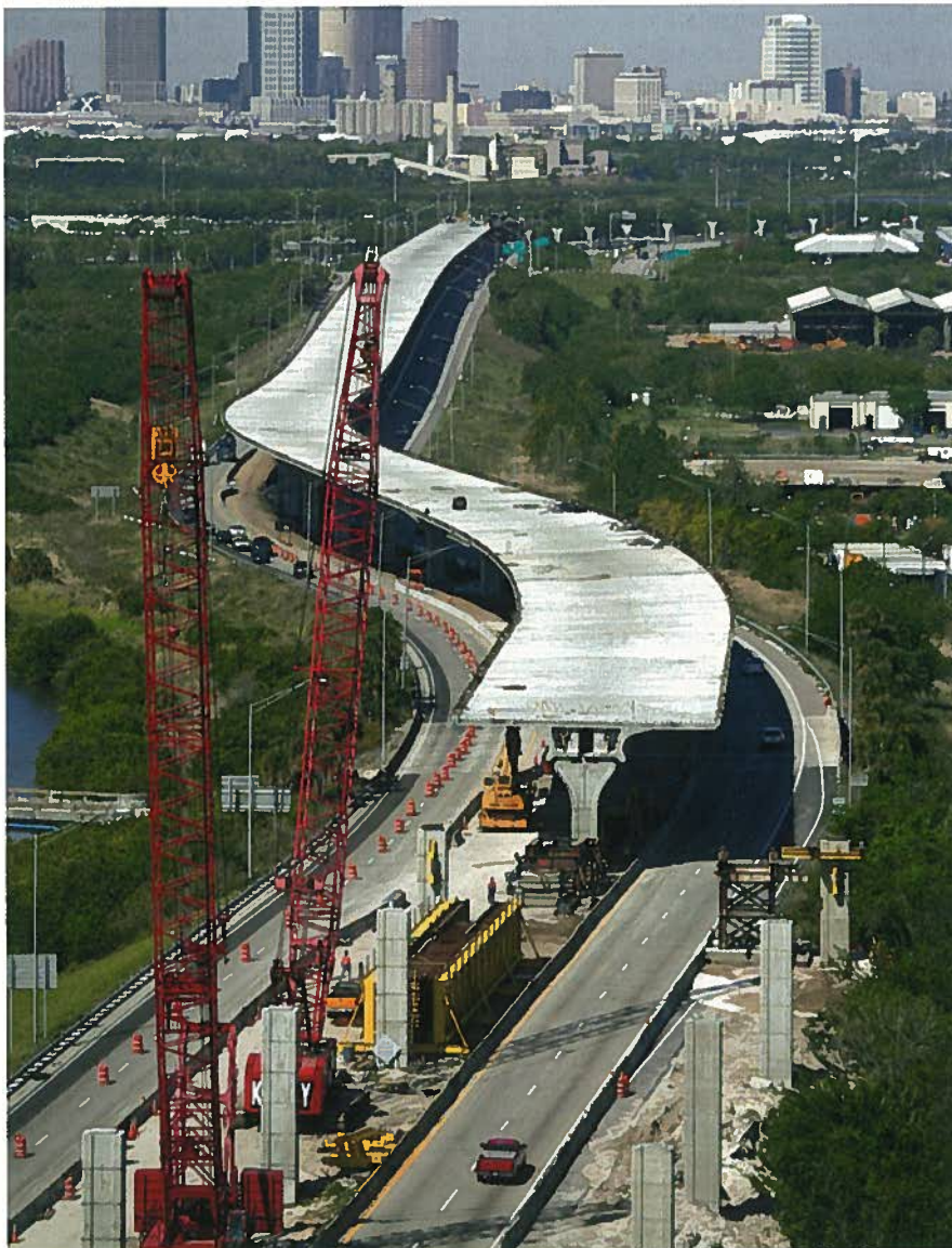
Fig. 1. Presently under construction over moving traffic, the Lee Roy Selmon Expressway in Tampa, Florida, supports six lanes of traffic on single piers only 6 ft (1.8 m) wide, and demonstrates the extraordinary evolution of precast concrete segmental bridges in the last thirty years.
