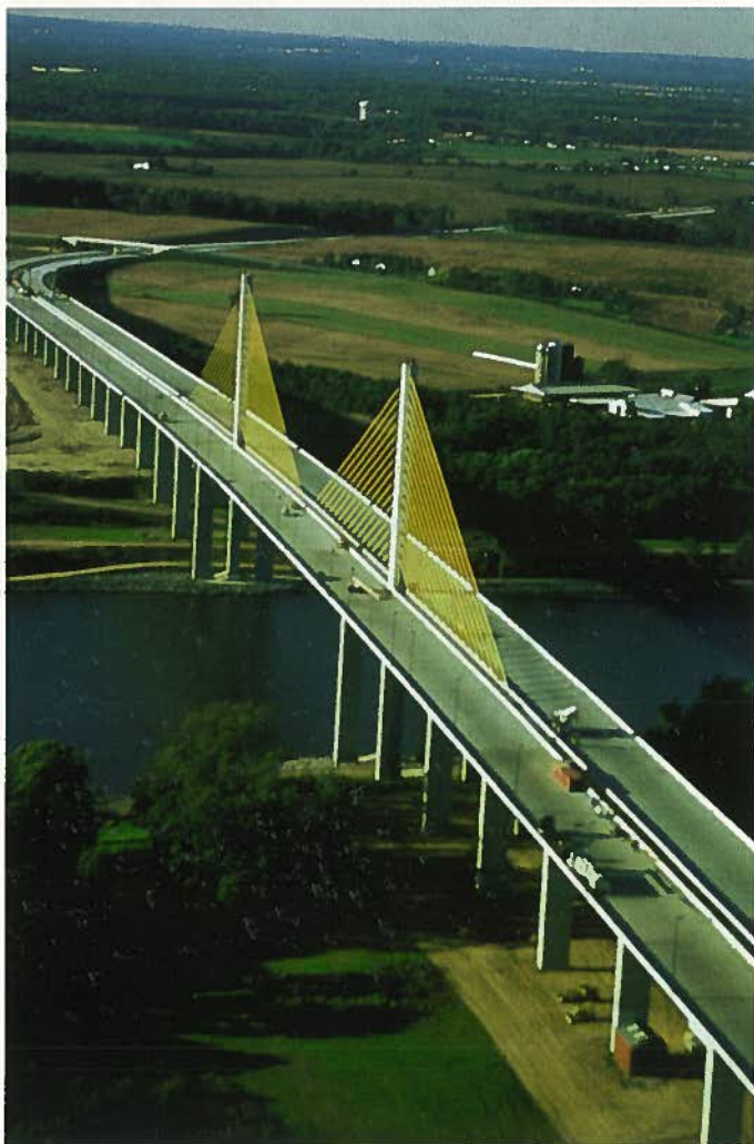
Fig. 19. Completed in 1995, the Chesapeake & Delaware Canal Bridge near St. Georges, Delaware, was the first precast concrete cable-stayed bridge in the northeast United States. Using innovative design solutions, including precast concrete delta frames, this bridge delivered a savings of $6.2 million over alternate bid designs.
