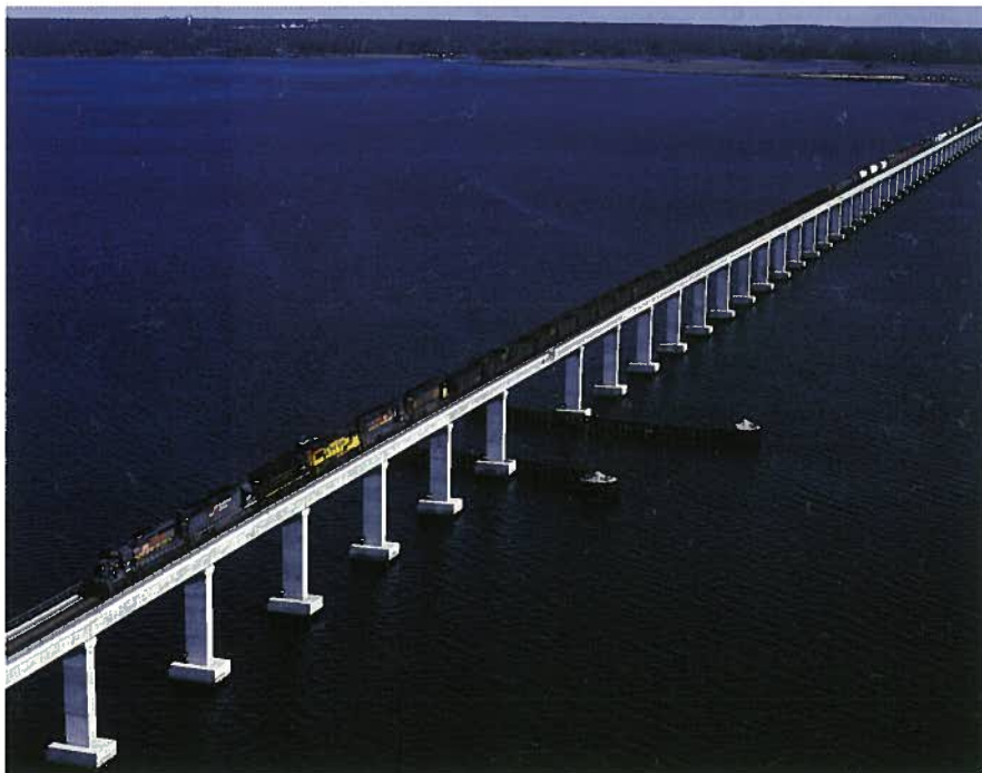
Fig. 18. The John T. Collinson Rail Bridge near Pensacola, Florida, is the first use of precast concrete segmental technology for a heavy rail bridge in North America. The bridge is designed to handle the heaviest train loadings, hurricane force winds, and barge impacts.
