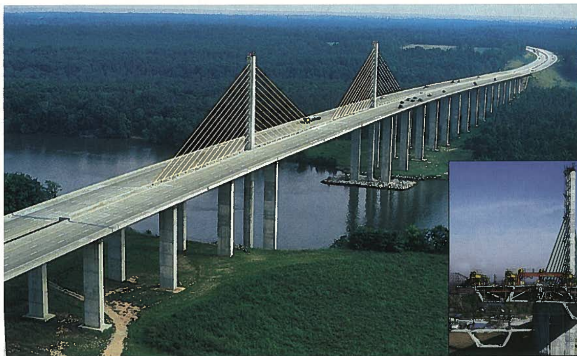
Fig. 8. The Varina-Enon Bridge near Richmond, Virginia, features the world's first use of precast concrete delta frames for construction of its 630 ft (192 m) cable-stayed main span. This elegant and durable structure sustained a direct tornado impact without damage.
