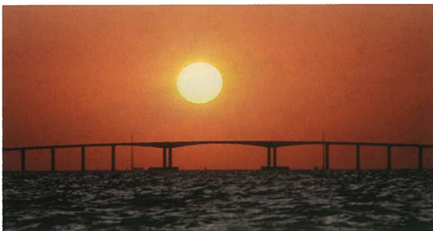
Fig. 7. The Dauphin Island Bridge in Mobile, Alabama, was built in just 34 months, featuring a 400 ft (122 m) main span – the longest precast concrete segmental span at the time of completion in 1982.
