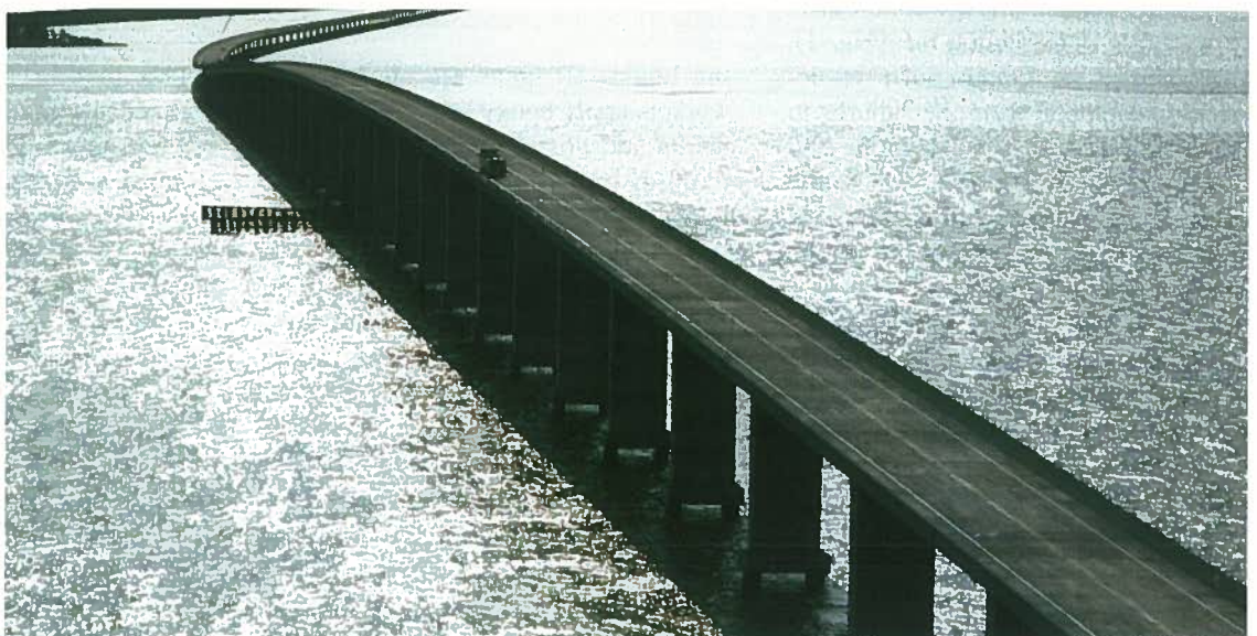
Fig. 3. The longest continuous precast segmental bridge in the world in 1982, the Seven Mile Bridge in the Florida Keys was the first use in North America of precast, match-cast box piers, assembled with vertical post-tensioning.
