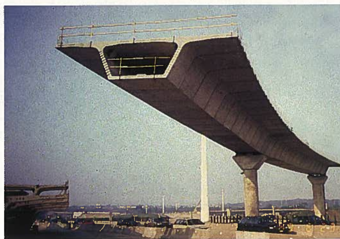
Fig. 13. The Illinois Tollway Interchange, near Chicago, Illinois, demonstrates that segmental concrete structures can be built over major traffic flows.
