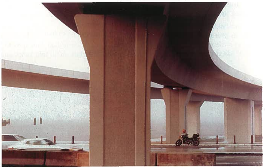
Fig. 11. Biloxi I-110 in Mississippi was built over the four-lane U.S. 90 to minimize traffic interruptions. $4.2 million was saved over the alternate construction system at the time of bidding.
