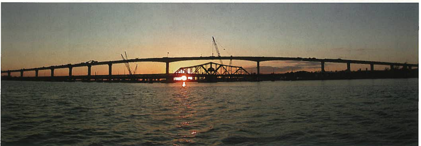
Fig. 10. The 440 ft (134 m) precast fully match-cast main span of the Victory Bridge in northern New Jersey was dedicated on June 5, 2004; the twin span is scheduled for completion in 2005.
