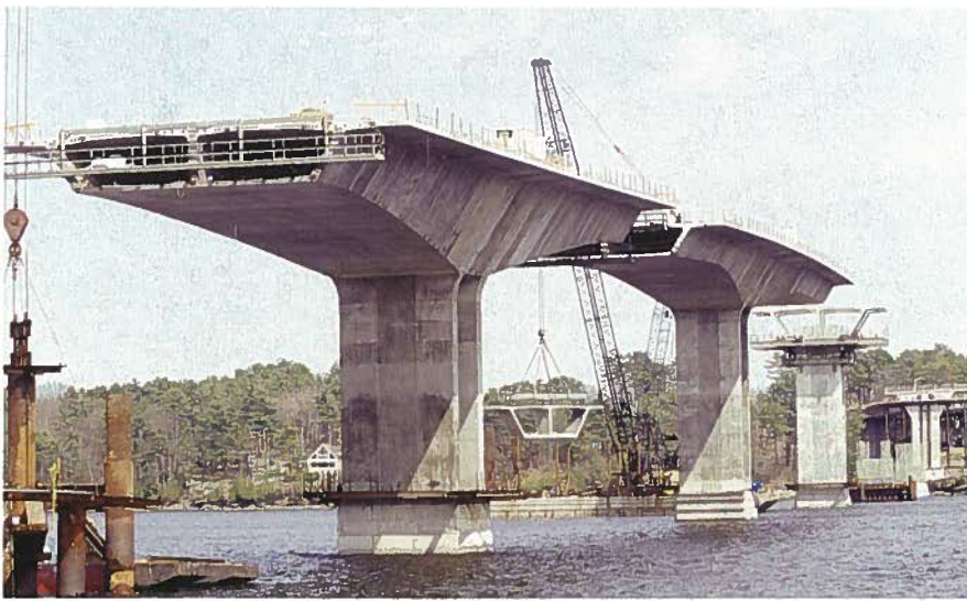
Fig. 9. Sagadahoc Bridge in Maine has a 420 ft (128 m) precast segmental main span and was completed in 2000. Precast concrete segments weighed 100 tons (91 tonnes).
