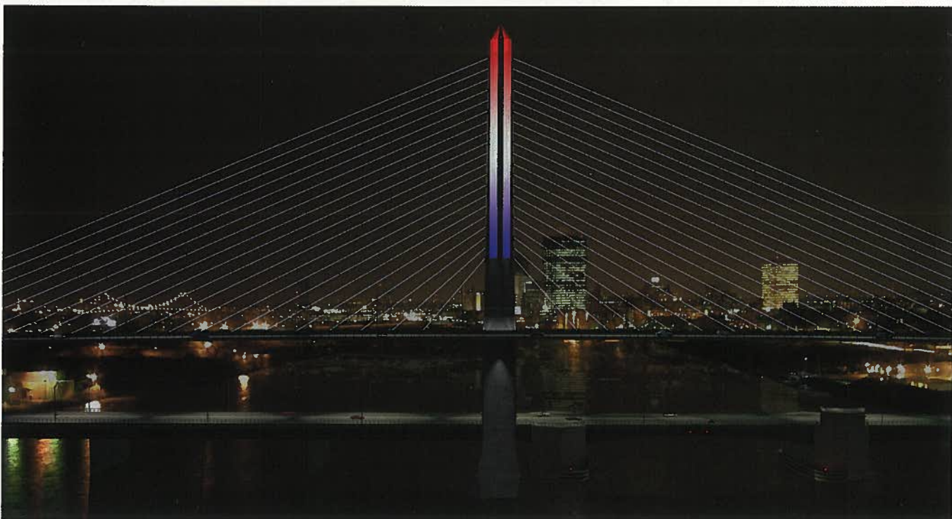
Fig. 15. Displaying patriotic colors, this dramatic night photo of the I-280 Maumee River Crossing in Ohio illuminates a new Toledo landmark. Specially engineered, the top 190 ft (57.9 m) of the single pylon is glass-clad, a community tribute to its glass industry. A first-of-its-kind cradle system carries the cable stays through the central pylon.
