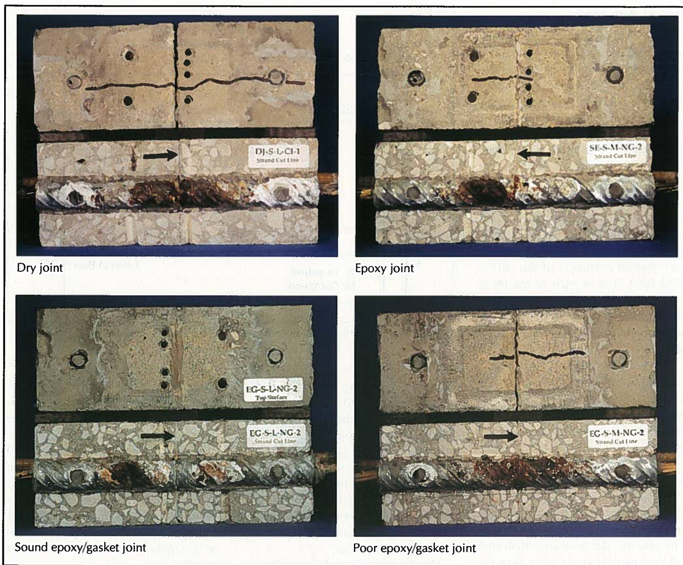
Fig. 16. Galvanized steel duct corrosion: effect of joint type.
