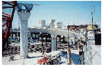
Fig. 11. Segmental concrete construction over North Station tracks.
