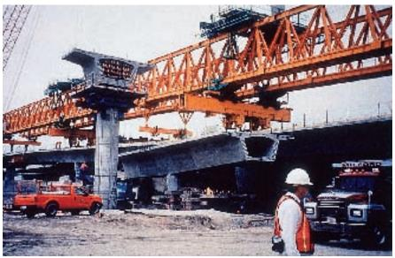
Fig. 3. Precast segmental erection.
