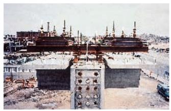
Fig. 4. Precast segments connection to straddle pier.
