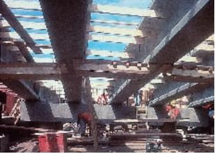
Fig. 12. New England bulb-tee girder construction.
