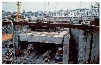
Fig. 5. Precast tunnel jacking.
