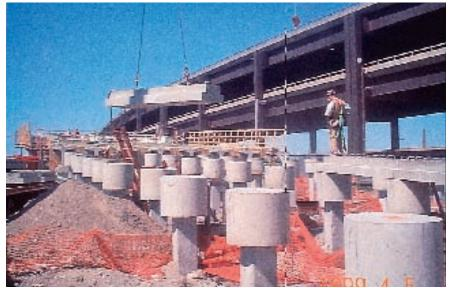
Fig. 13. Slab-on-pile erection.
