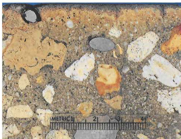
Note the presence of cracks in the region of pink discoloration. Also observe the partial change of aggregate color (upper right) from yellow gold to red.
