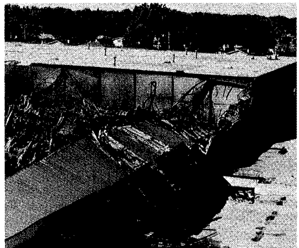
Fire at Montgomery Ward warehouse, Bensenville, Illinois. Photo courtesy of National Fire Protection Association.
