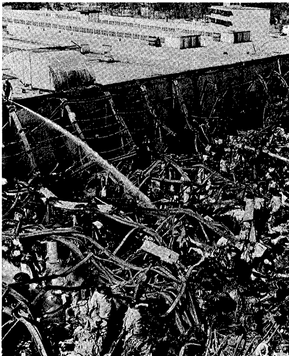
A properly constructed firewall with adequately protected openings can stop a fire from spreading even when automatic and manual firefighting efforts have failed.
