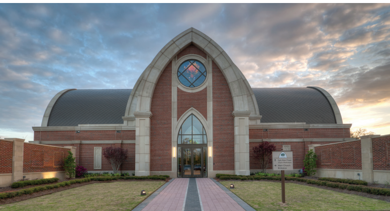
St. George Catholic Church in Baton Rouge, La., used load-bearing precast concrete panels from Gate Precast to eliminate much of the steel specified in the original design. Courtesy of www.toddlandryphotography.com .
