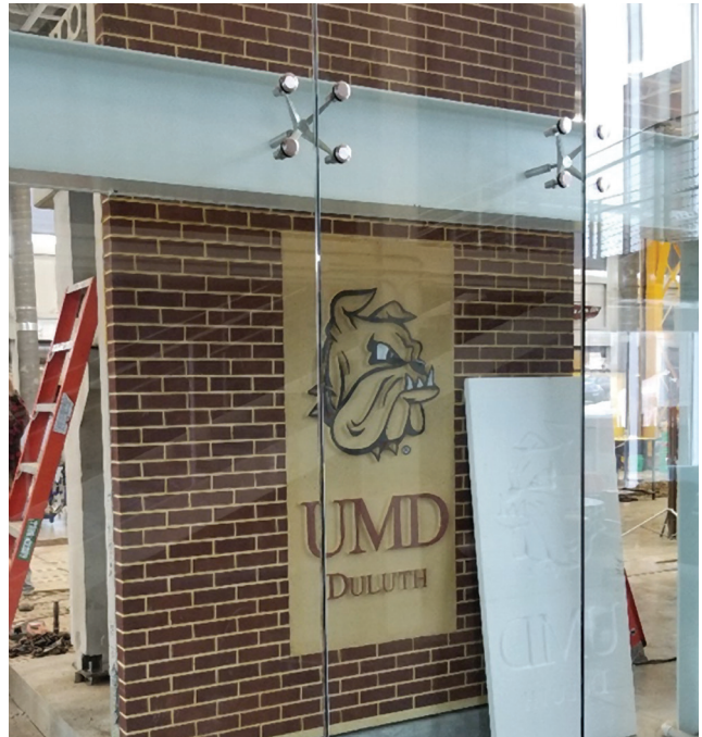
The front view of the completed precast concrete demonstration structure in the University of Minnesota Duluth (UMD) teaching high bay laboratory shows the UMD Bulldog logo, which was cast face down in the form with a gold-colored architectural concrete mixture, and thin brick. Courtesy of Ben Dymond.
