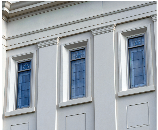
The Cedar City Temple’s precast concrete panels provide fine detail that would be expensive to achieve in stone because the detail would need to be hand chiseled. Courtesy of Juan R. Sanchez/Forterra.
