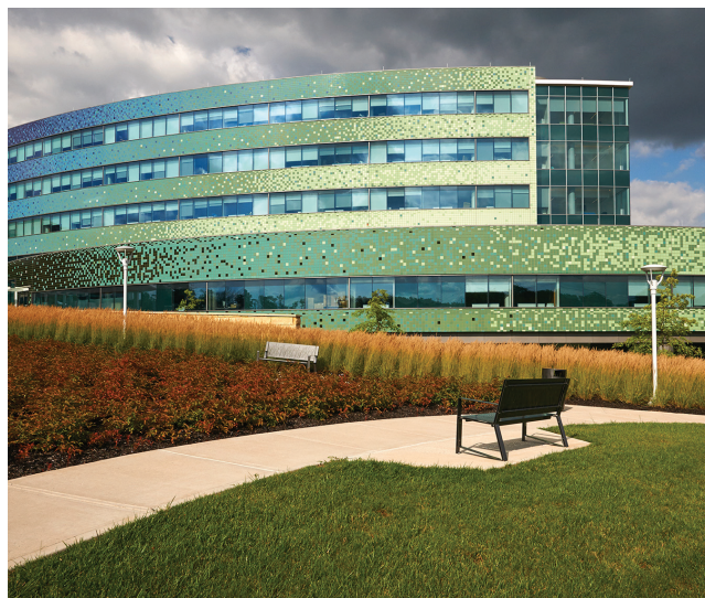
The Mercy Health–West Hospital in Cincinnati, Ohio, used insulated sandwich panels to provide energy efficiency and span from column to column. Courtesy of Nathan Cox.
