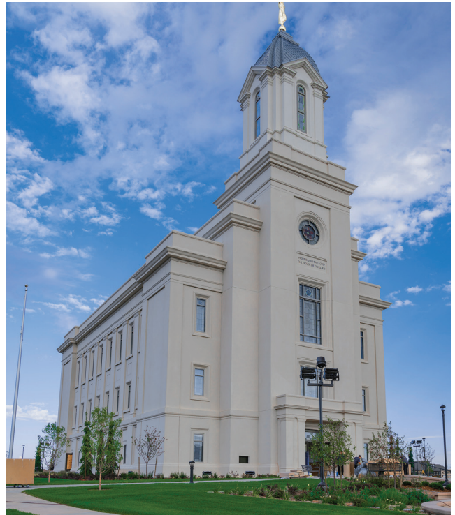
The Cedar City Temple of the Church of Jesus Christ of Latter-day Saints (LDS) in Utah uses reinforced, architecturally finished precast concrete panels on the majority of the temple and glass-fiber-reinforced concrete panels on the spires and a few other locations. Courtesy of Juan R. Sanchez/Forterra.
