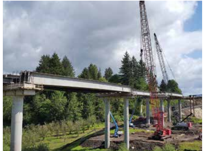
Cranes lifted precast concrete girders into place for the Chehalem Creek Bridge. Courtesy of the Oregon Department of Transportation.
