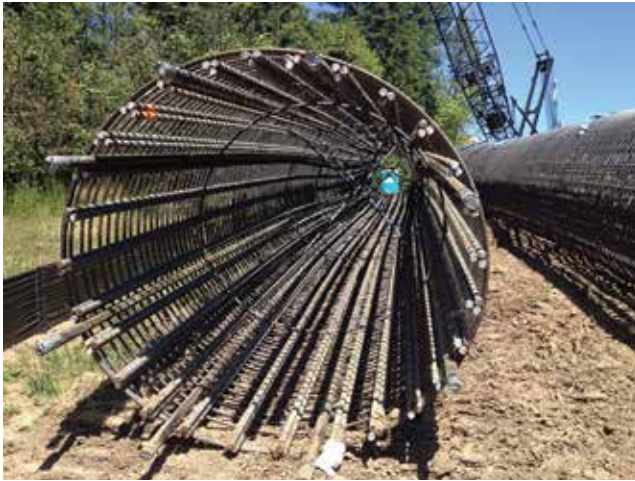
This reinforcement cage was used in the construction of a drilled shaft for the Chehalem Creek Bridge in Yamhill County. Courtesy of the Oregon Department of Transportation.
