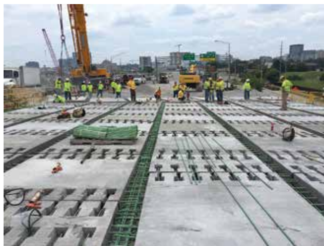
Workers place epoxy-coated steel reinforcing bars into a section of Interstate 40 for the Fast Fix 8 project in Tennessee. Courtesy of Gresham, Smith & Partners.
