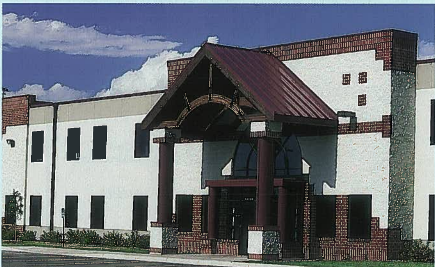
Schwieters Construction Park, Hugo, Minnesota. The project utilizes Fabcon's insulated loadbearing panels for maximized energy efficiency of the facility.
