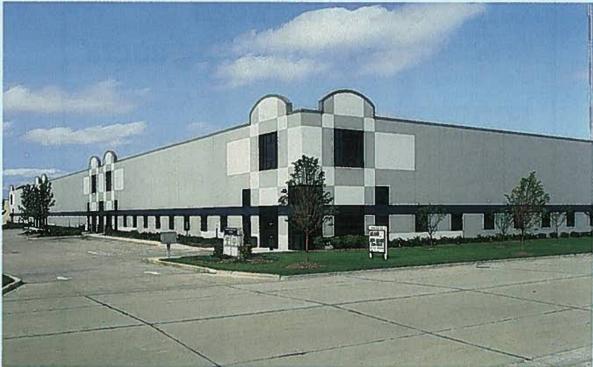
Glendale Commerce Center, Glendale, Wisconsin. This structure displays the widest spectrum of finishes, aggregates, patterns, tints, graphics and decorative banding offered by Fabcon.
