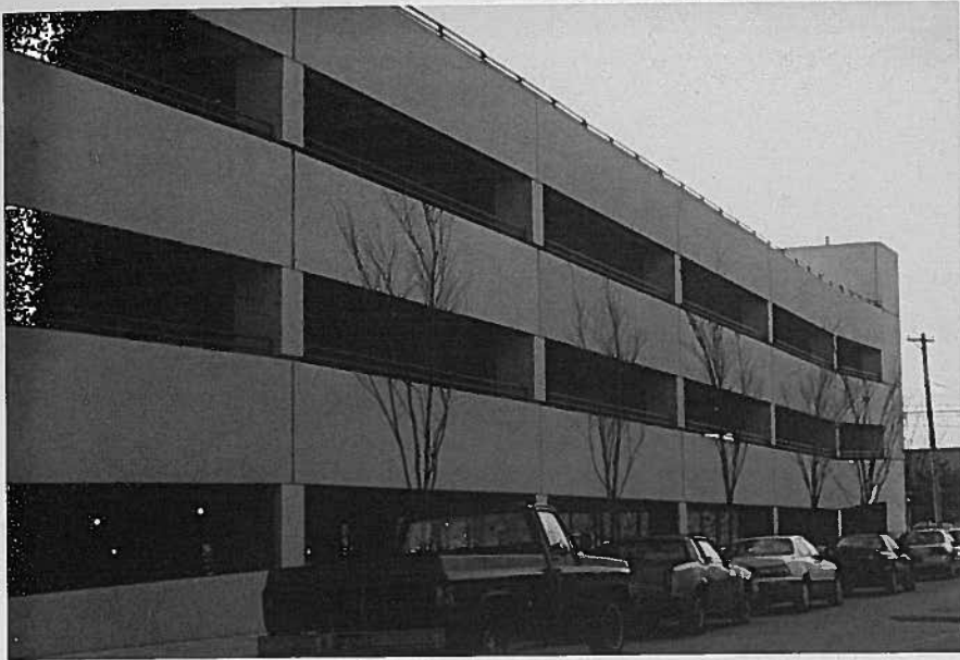
The new parking garage for Delaware Technical and Community College in Wilmington, Delaware.
