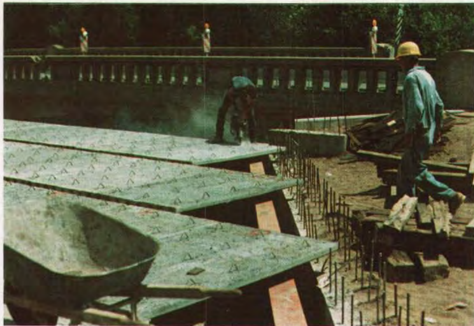
Fig. B7. A three span wide flange steel beam bridge over a stream near Peoria, Illinois. The panels were made rectangular and cut in the field to fit the skew.
