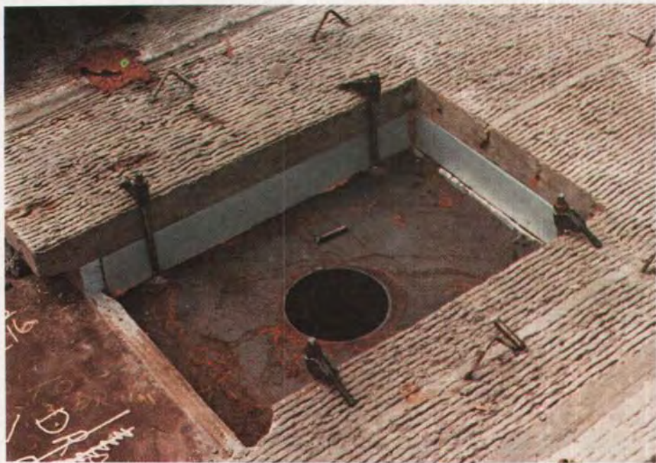
Fig. B4. The blockout for a scupper.
