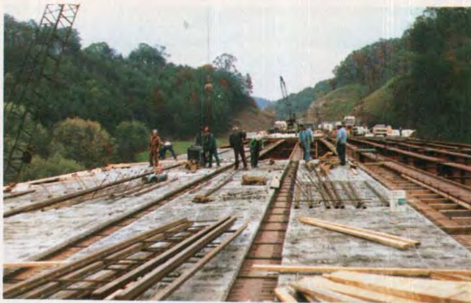
Fig. 2. Welded steel plate girder stream crossing in eastern Kentucky used the detail shown below. The steel frames are fabricated on site after determining the height from top of flange (bottom of 2 in. bar) to bottom of deck (top of angle).
