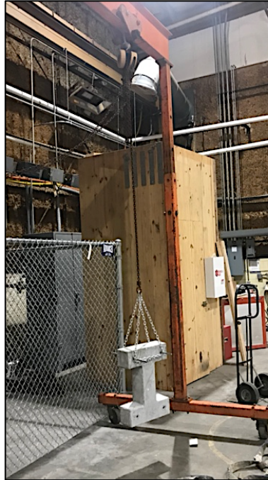
Figure 11: Lifting strategy for tiles using chain hoist.
