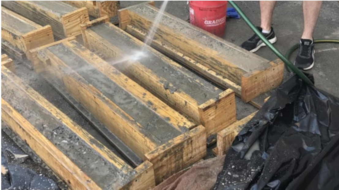
Fig. 4 Preparing the exposed aggregate surface on the HSFRC laminate face.
