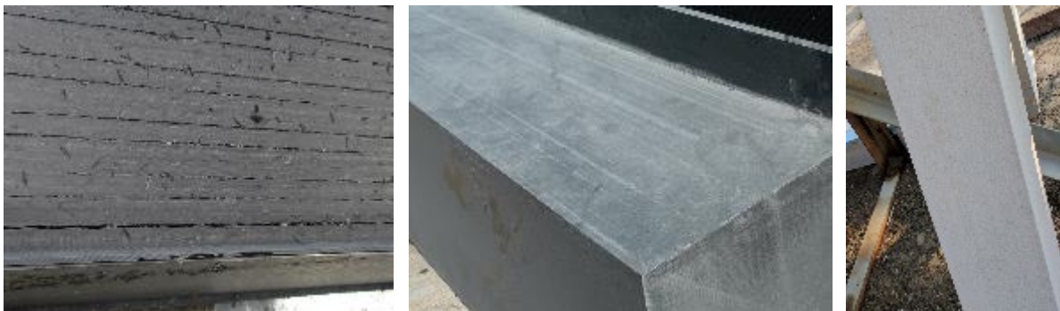
Figure 27. Left: horizontal surface of north mold after machining showed large voids between layers. Middle: voids were filled with 2-part epoxy. Right: voids reopened and bleeding of concrete in the voids caused dark lines in the concrete.
