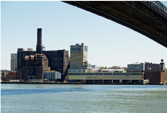
Figure 1. Domino Factory as viewed from the water under the Williamsburg Bridge prior to selected demolition. Photo by David Shankbone/Wikimedia Commons ( https://commons.wikimedia.org/wiki/File:Domino_Sugar_Williamsburg_New_York_by_David_Shankbone.jpg )
