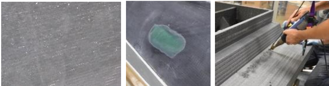
Figure 30. Left: small gaps that emerged between the printed layers and got filled with concrete did not affect the finish of the concrete parts. Middle and right: dents and larger gaps were fixed with a fiberglass reinforced filler or ABS that was applied with a “welding gun”.
