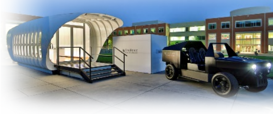
Figure 4. 3D printed Additive Manufactured Integrated Energy (AMIE), which connected a natural-gas-powered hybrid electric vehicle to a high-performance building that produces, consumes, and stores renewable energy.
