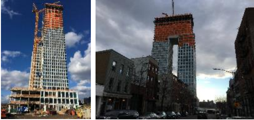
Figure 33. Construction progress as of March, 2019
