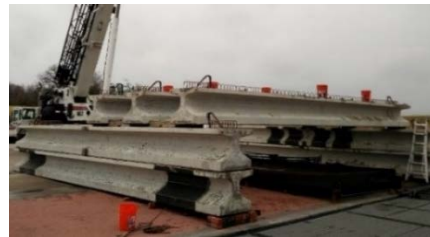
(b) supports and girders after placement
