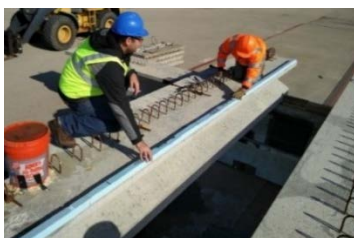
(c) bedding strip installation
