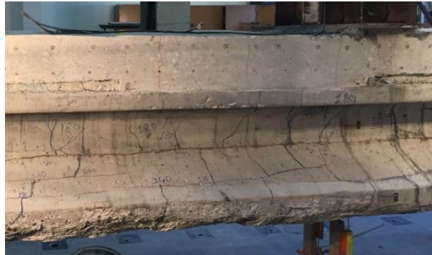
(b) crack patterns
