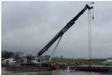
(a) placing of support girders
