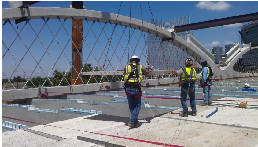
Fig. 1. Placement of precast prestressed concrete deck panels
