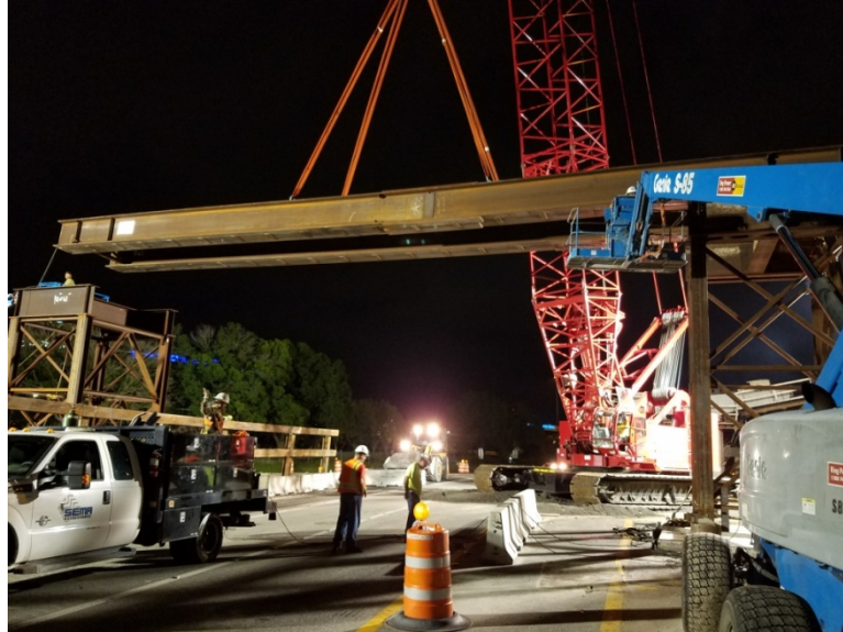
Fig. 6: Erecting Temporary Straddle Bent Over SR-202
