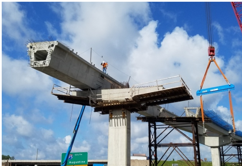
Fig. 4: Precast Pier Cap Supports Pier Girder During Construction
