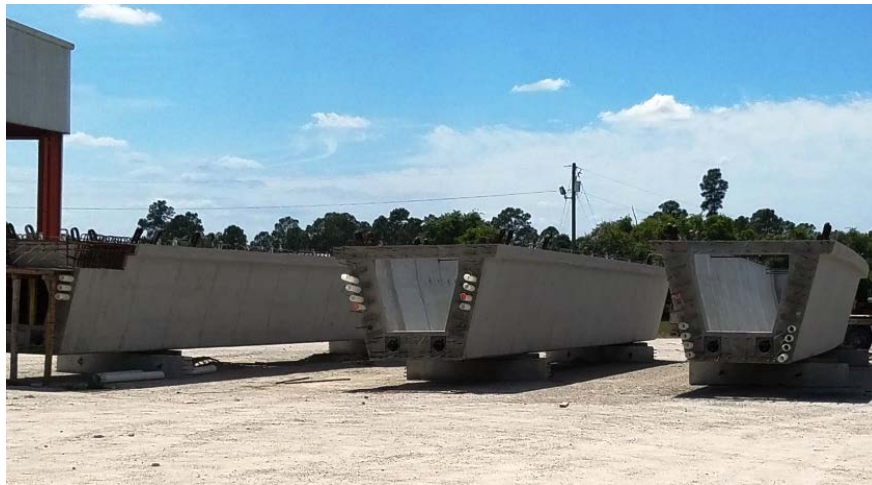
Fig. 13: Precast Girders in Storage
