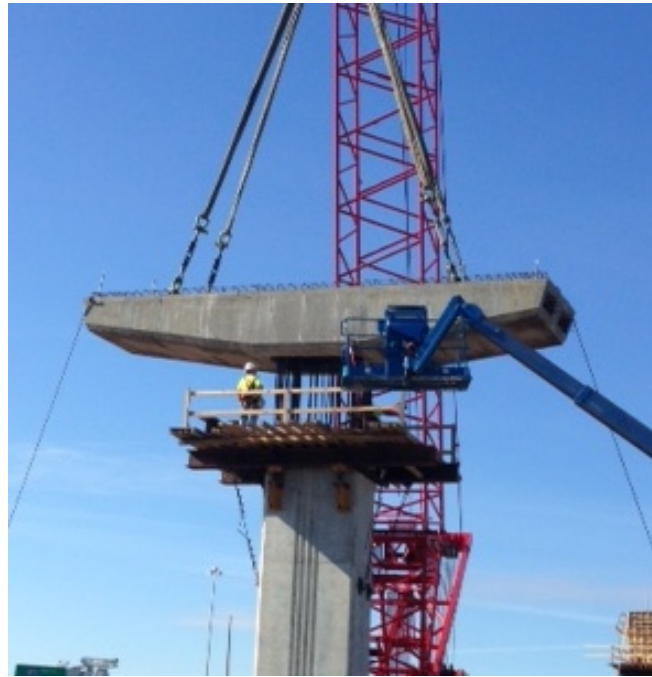
Fig. 3: Precast Pier Cap Erected onto Temporary Falsework
