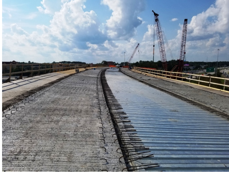
Fig. 17: CIP Lid Slabs Cast in the Field
