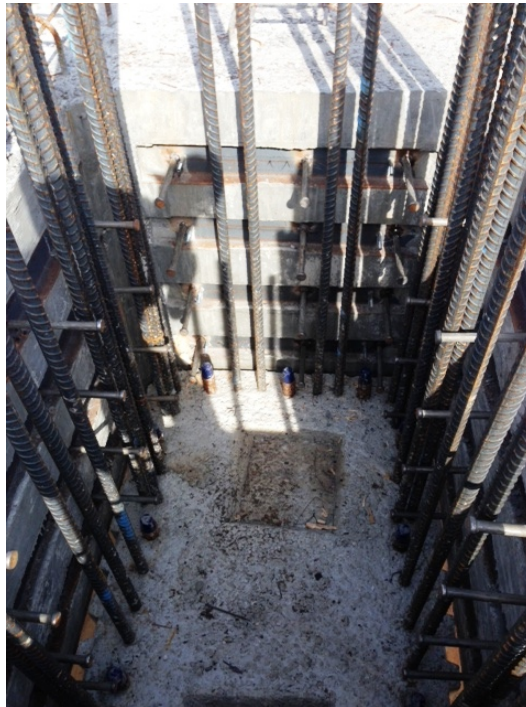
Fig. 10: Column-To-Cap Connection.
