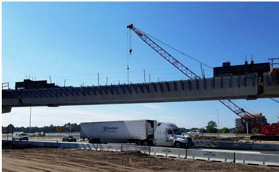
Fig 19: Precast Girders Supported on Strongbacks
