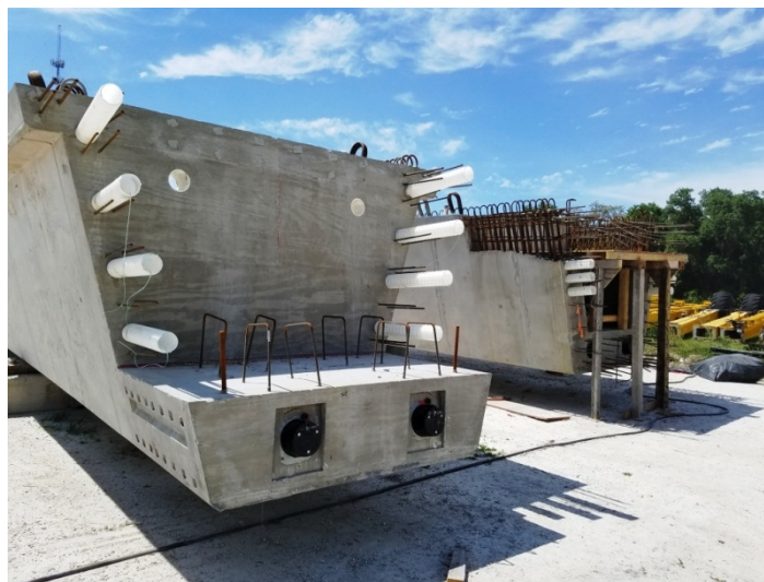
Fig. 15: Tongue Section at End Girder
