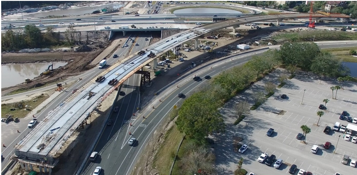
Fig 1: Flyover Bridge During Construction
