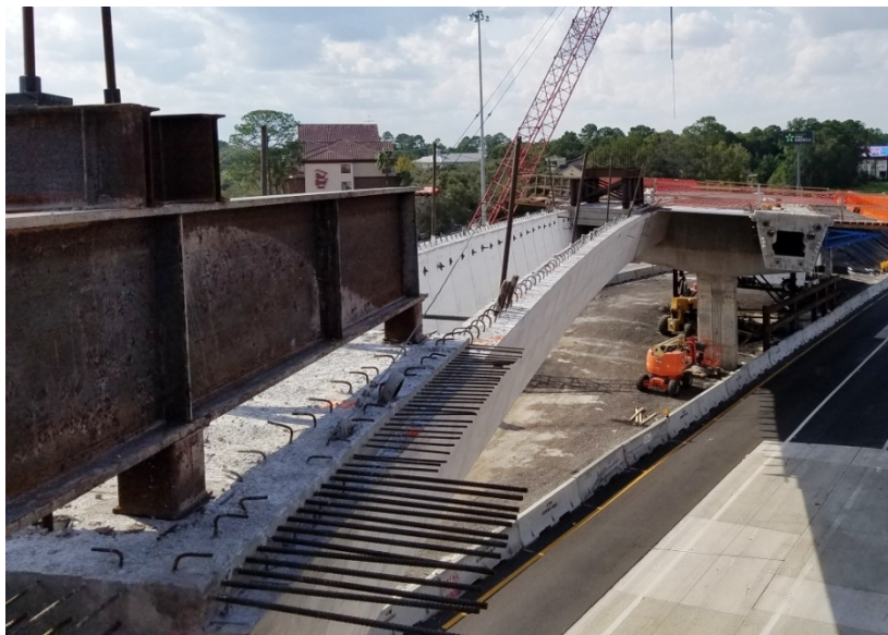
Fig. 5: Drop-in Girder Supported on Strongbacks Over I-95
