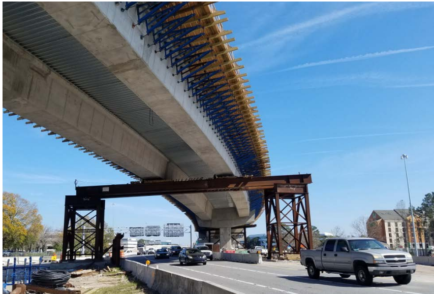
Fig. 16: Precast Girders Supported on Straddle Bent Over SR-202
