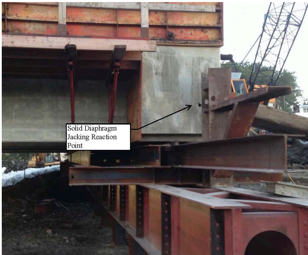
Figure 5 – Massena Solid Diaphragm Jacking Reaction Point
