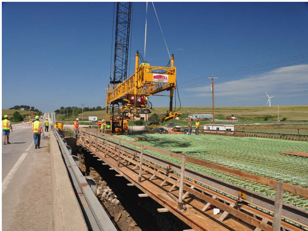
Figure 1 – Constructing New Massena Bridge
