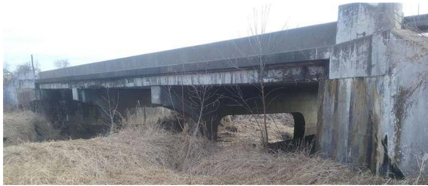
Figure 3 – Existing IA 1 Bridge over Camp Creek
