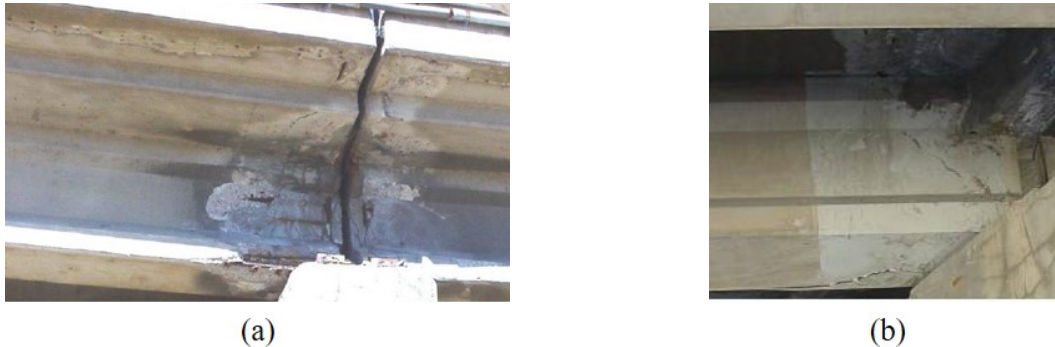
61 Fig. 1 End region of prestressed girder: (a) end damage of girder; (b) typical mortar repair of 62 girder end 63
