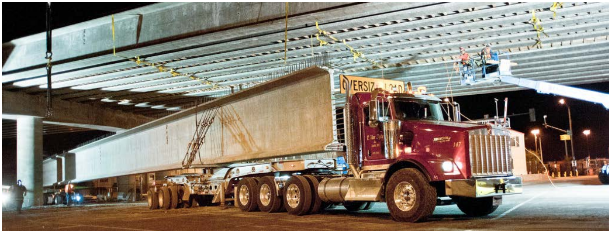
Figure 3 - Transport of 205 ft, WF100G Girder
