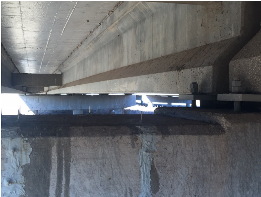
Figure 2. View underneath the North Canadian Overflow Structure. John Kilpatrick Turnpike, Oklahoma.
