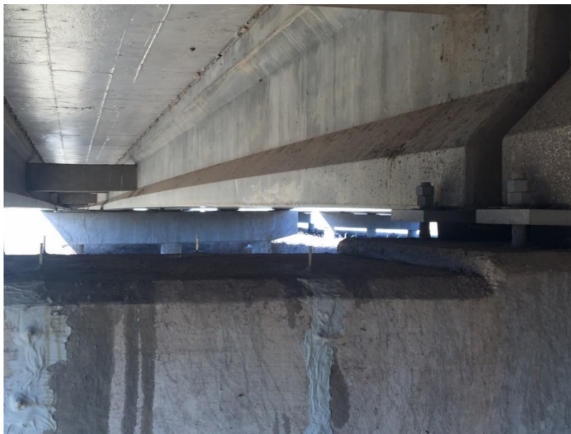
Figure 2. View underneath the North Canadian Overflow Structure. John Kilpatrick Turnpike, Oklahoma.
