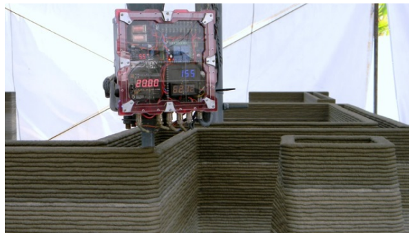
104 Fig. 3- 3-D printing of concrete (photo courtesy of 3D Concrete House Printer 6 , used with 105 permission)
