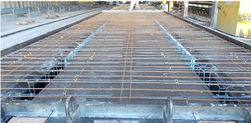
Fig. 10. FVDT prior to casting
