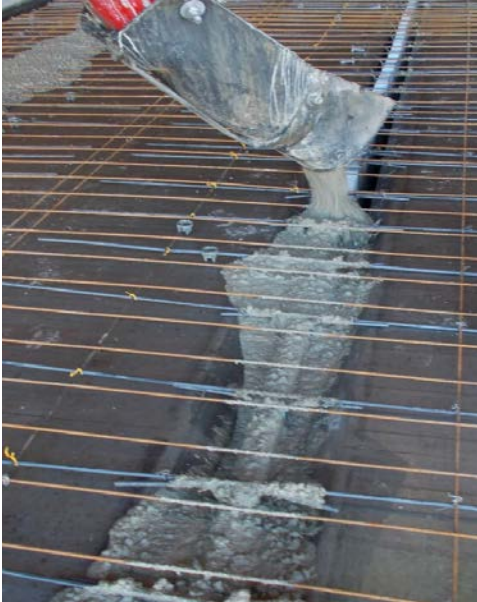
Fig. 11. Concrete placement in stem
