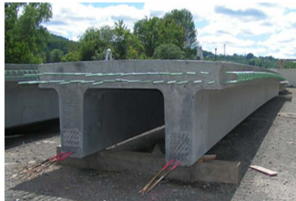
79 80 Fig. 3. Early DT (left, figure from Edwards) and NEXT beams (right, photo from L. C. 81 Whitford Materials Co., Inc.)
