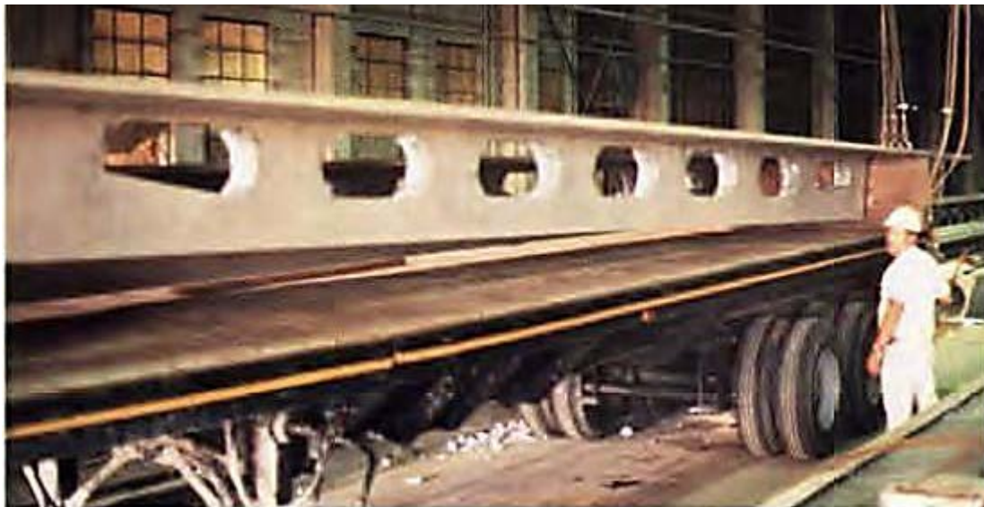
106 107 Fig. 5. Single tee with web openings (photo courtesy- M. Tadros 5 )
