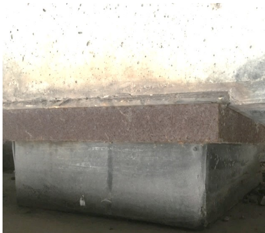
Fig. 6 Bearing rotation at the obtuse corner (Source: John Bolka, WisDOT).
