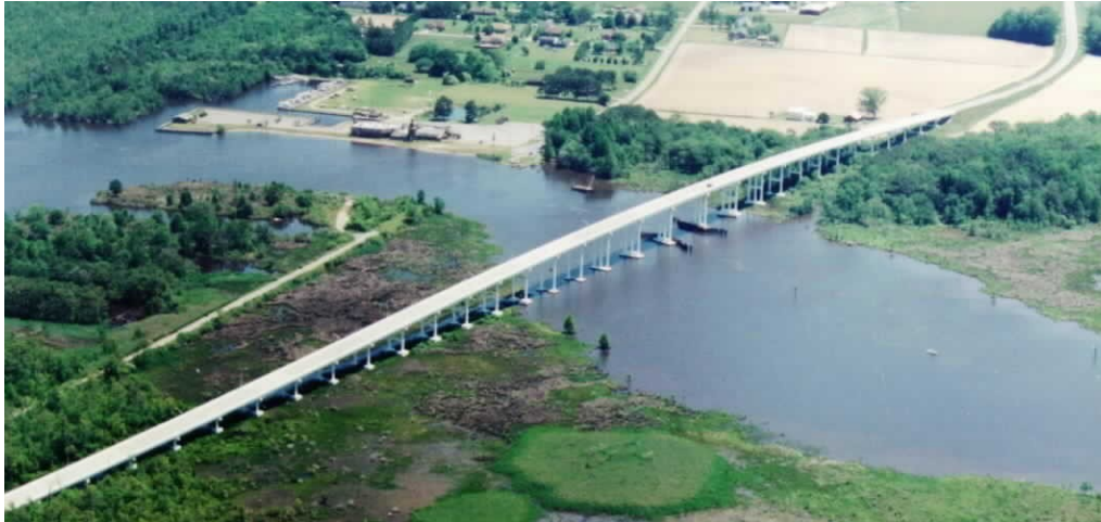
Fig. 6 Photograph of the Pungo Ferry Road Bridge shortly after completion
