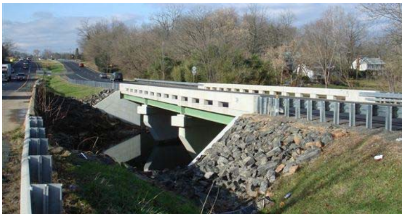
Fig. 14 Completed U.S. 15/29 bridge over Broad Run, looking South 13
