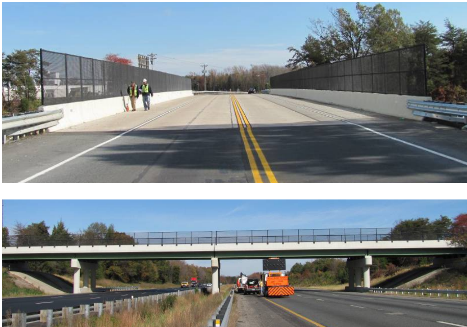
Fig. 8 Photos of completed Massaponax Church Road (Route 608) Bridge over Interstate 95 (VDOT)
