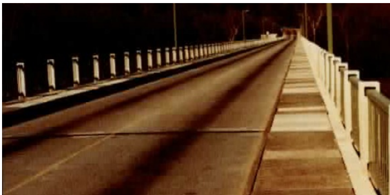
Fig. 1 Photograph of the Boulevard Bridge deck in 1983, after 24 years in service.
