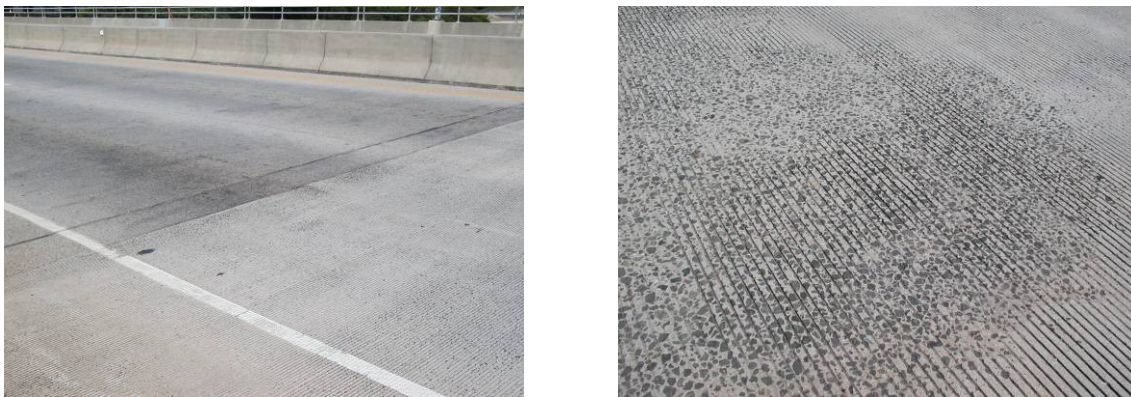
Fig. 12 Lightweight concrete deck on truss spans of the Coleman Bridge
