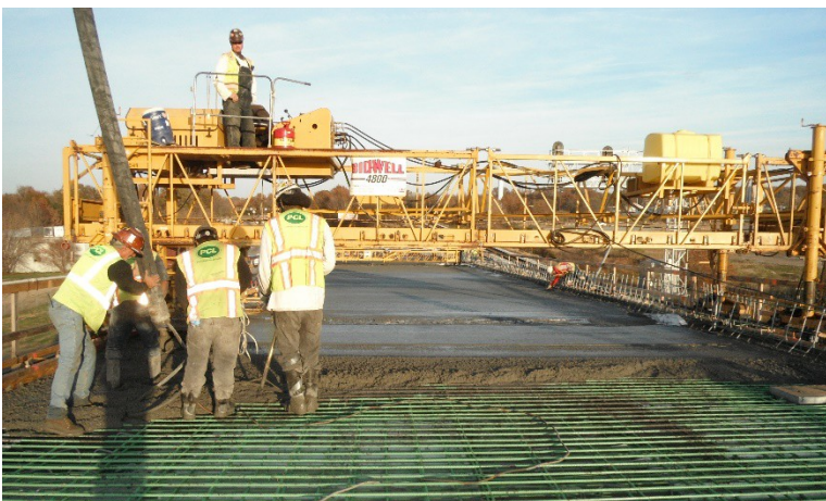
Fig. 10 Lightweight concrete being placed on new Gilmerton Bridge (PCL)
