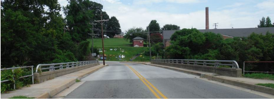
Fig. 4 Photograph of the Route 36 Bridge over Appomattox River (VDOT)
