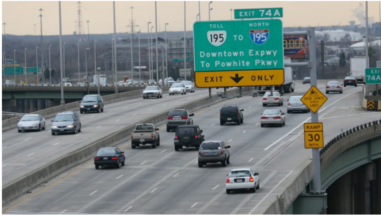
Fig. 13 Completed I-95 Bridge over the James River
