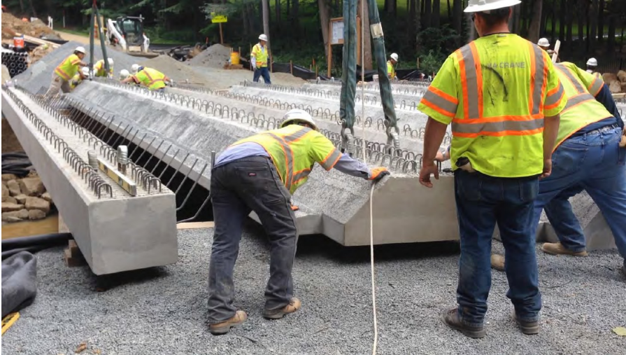
Fig. 21 Erection photo of inverted tee beams 20
