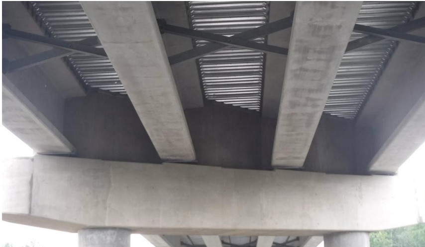
Fig. 19 Completed Route 17 Bridge from beneath (VDOT)
