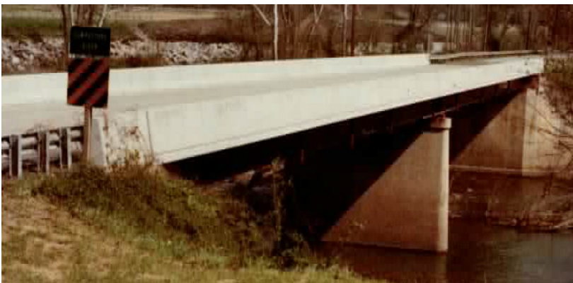
Fig. 5 Photograph of the Cowpasture Bridge in 1983
