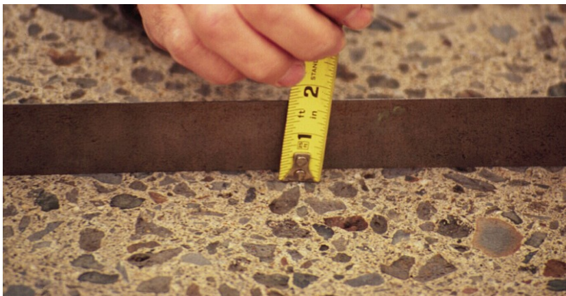
Fig. 3 Close-up photograph of deck from the Boulevard Bridge in 1993.
