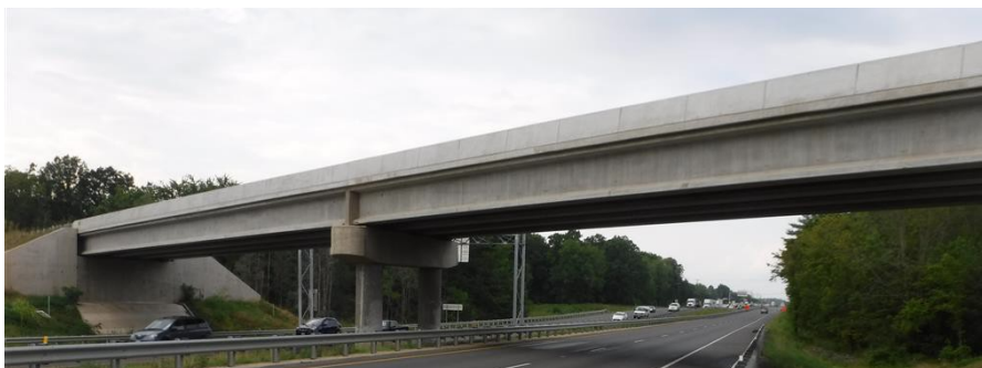
Fig. 18 Completed Route 17 Bridge (VDOT)
