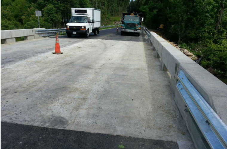
Fig. 22 Route 198 Bridge nearing completion
