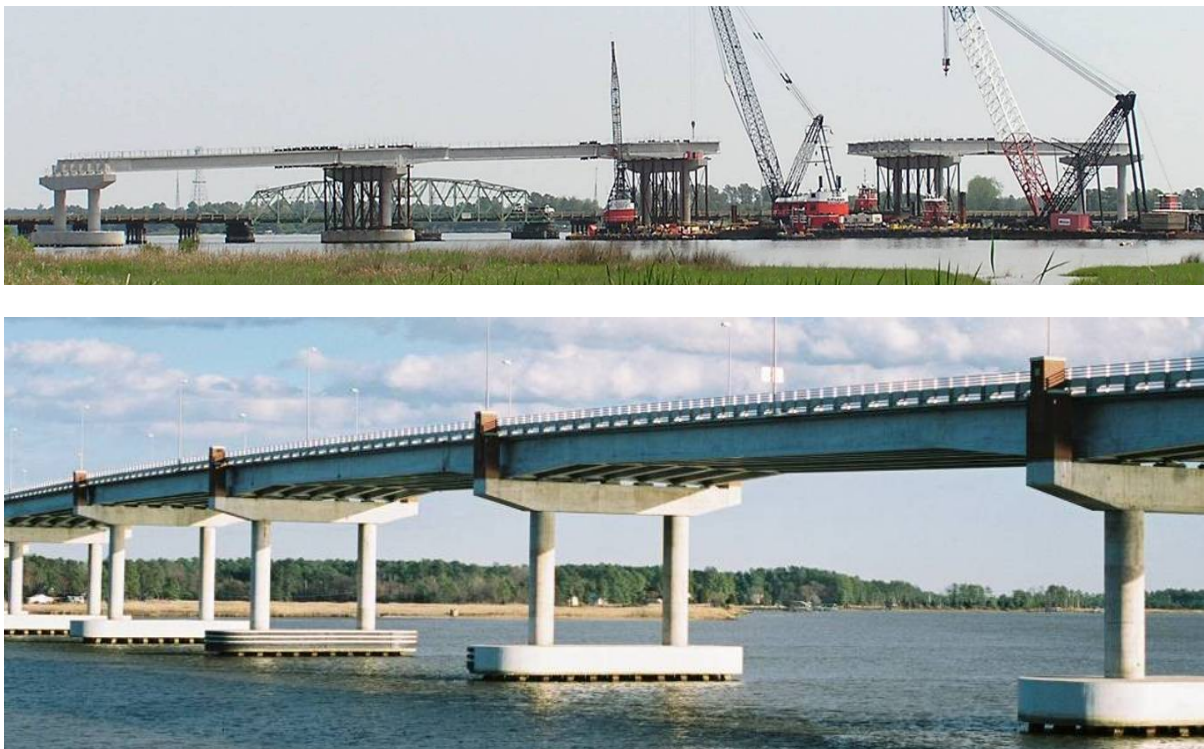
Fig. 16 Route 33 Bridge over the Mattaponi River under construction and completed
