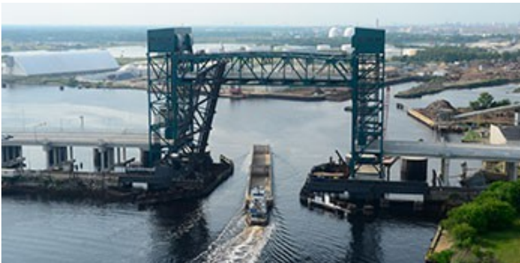
Fig. 9 The new Gilmerton Bridge (City of Chesapeake, VA)
