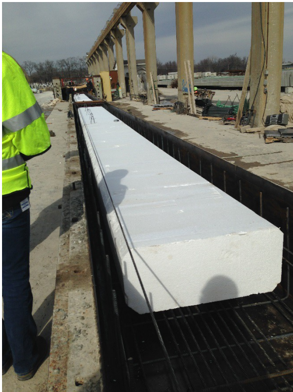
Figure 7 – Polystyrene Void in Precast Bed
