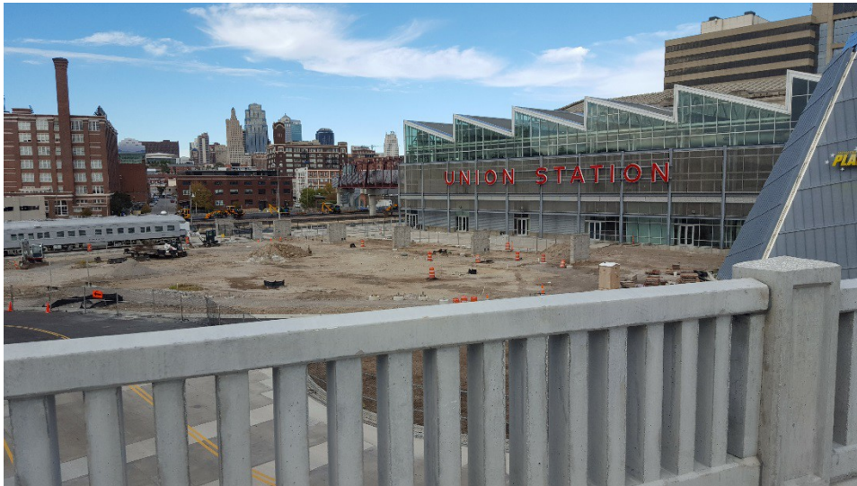
Figure 2 – New Ramp Bridge overlooking downtown Kansas City
