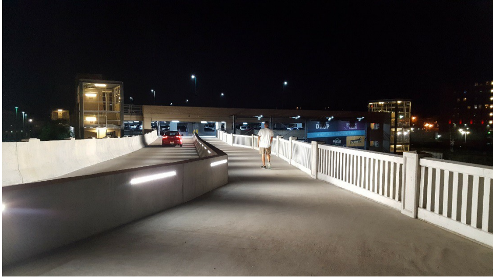
Figure 19 – New Bridge with Lighting
