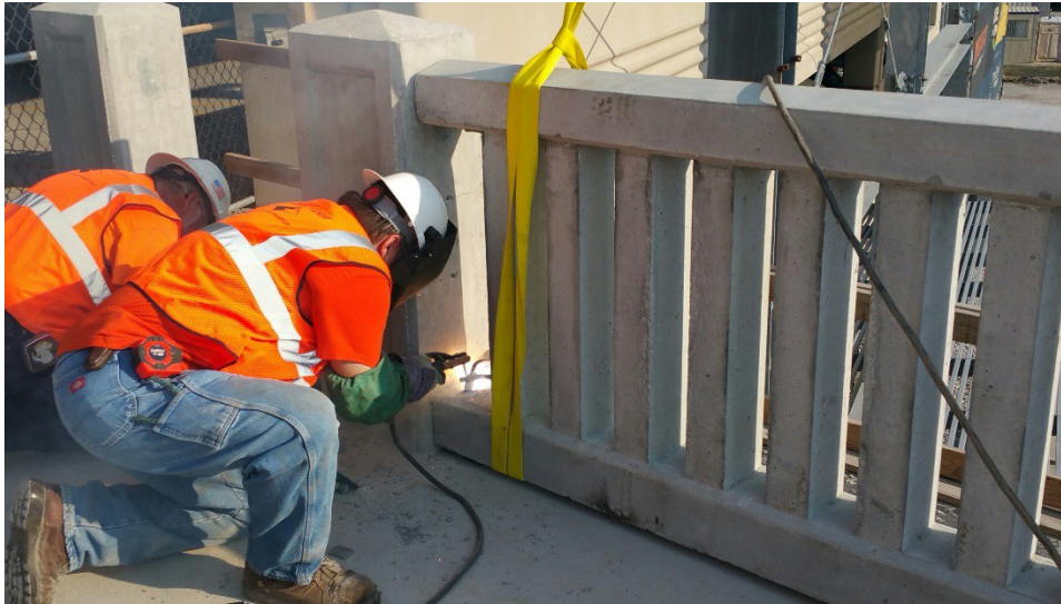
Figure 14 – Welded Connections for Precast Rail Panel
