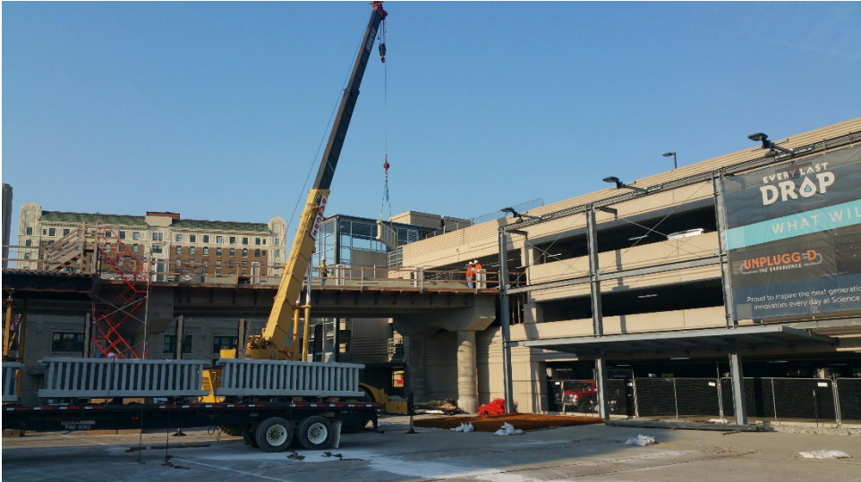
Figure 13 – Precast Rail Panel Erection
