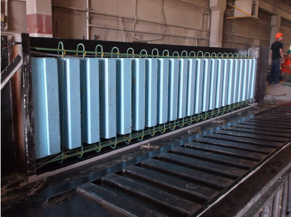
Figure 12 – Precast Rail Panel Formwork
