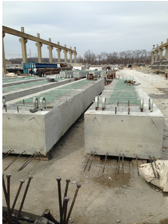
Figure 8 – Box Beams Awaiting Delivery
