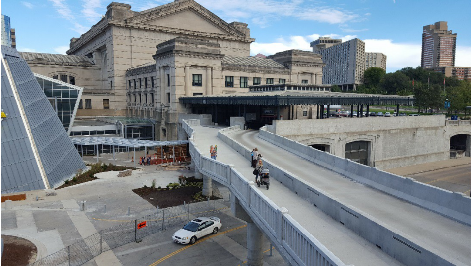
Figure 18 – New Bridge at Carriage Pavilion
