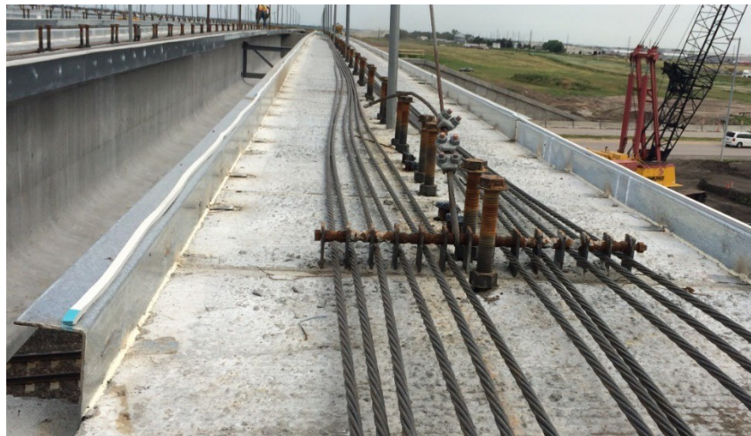
Figure 7: Deck support system and post-tensioning strands.
