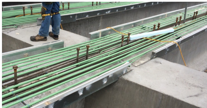
Figure 8: Live load continuity reinforcement over intermediate support.
