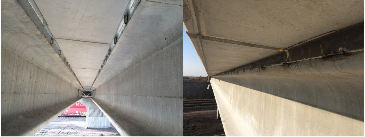
Figure 15: Bottom of precast concrete deck: between girders (a), and at the overhang (b)
