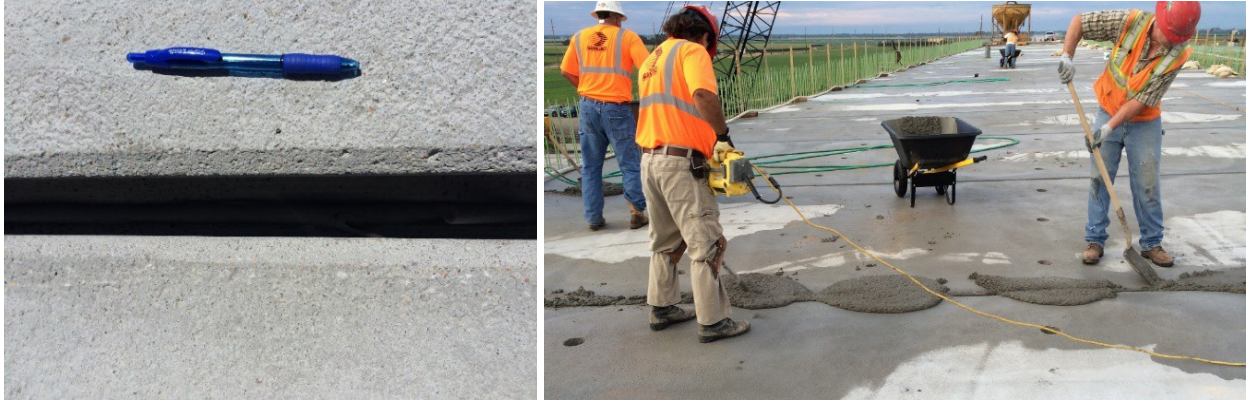
(a) (b) Figure 11: Placing concrete for transverse joints.
