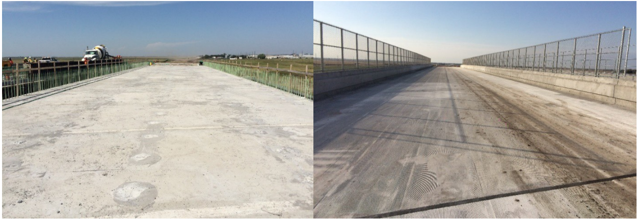
Figure 14: Final deck surface: before grinding (a), and after grinding (b)
