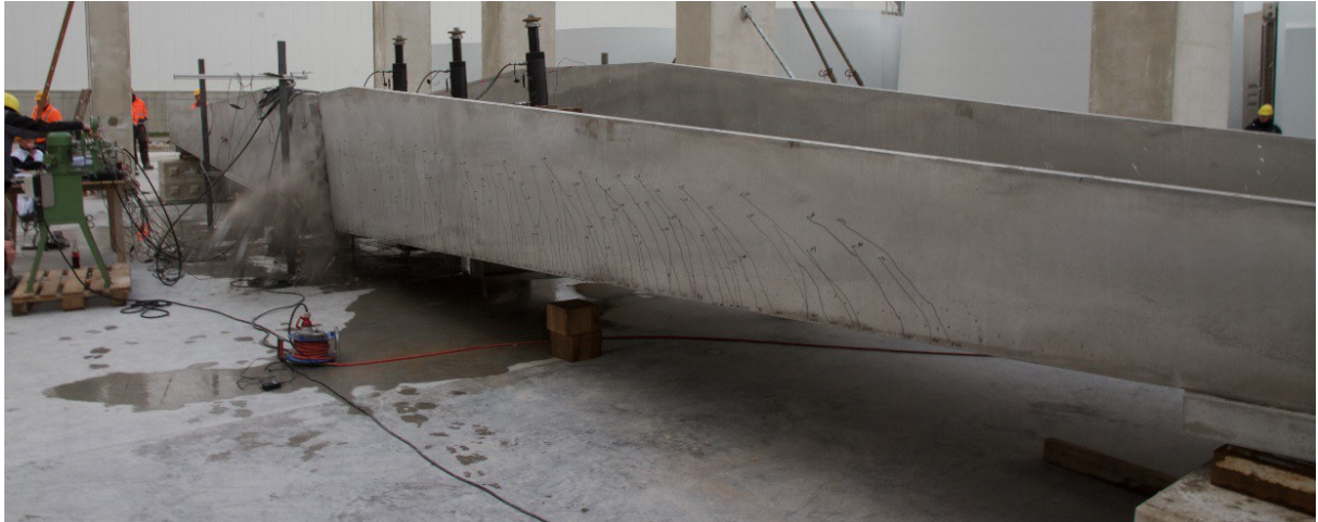
Fig. 21: View of the breaking point during the breaking process
