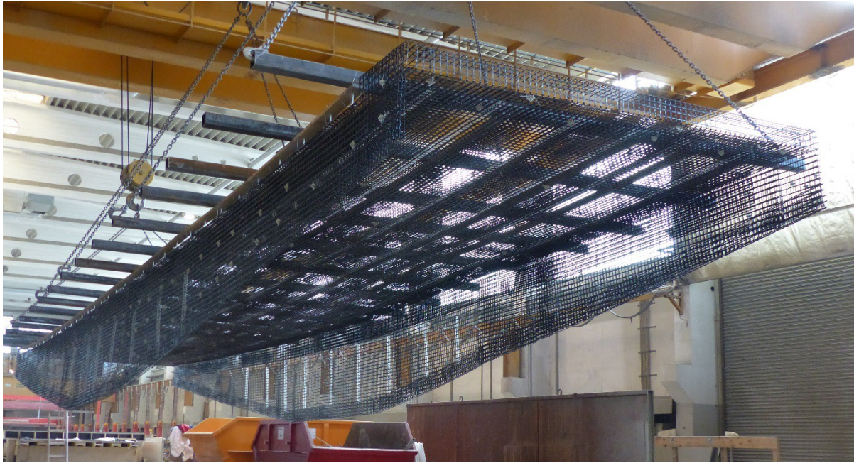
Fig. 6: Finished cage of reinforcement on the way into the formwork
