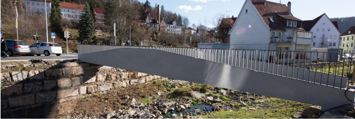
Fig. 1: TRC pedestrian Bridge in Albstadt, Germany (picture: solidian)
