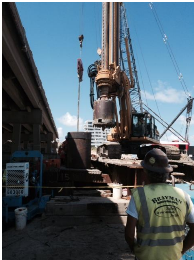
Figure 2- Drilled Shaft Drilling Bucket
