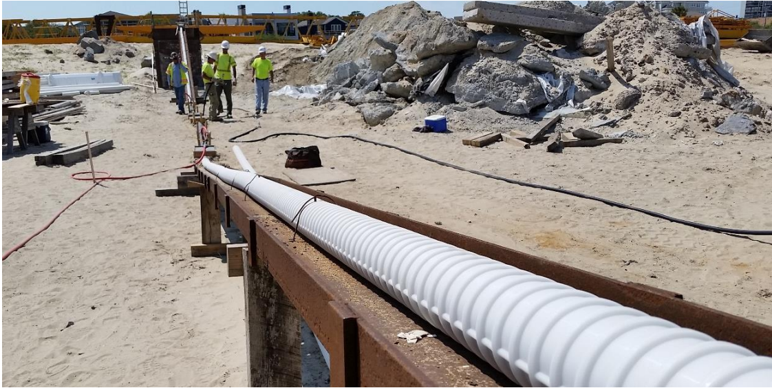
Figure 11 - Grouting Mock-Up
