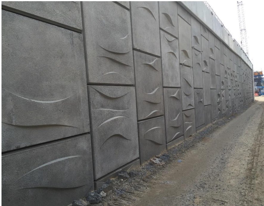
Figure 13 – MSE wall pre-cast panels
