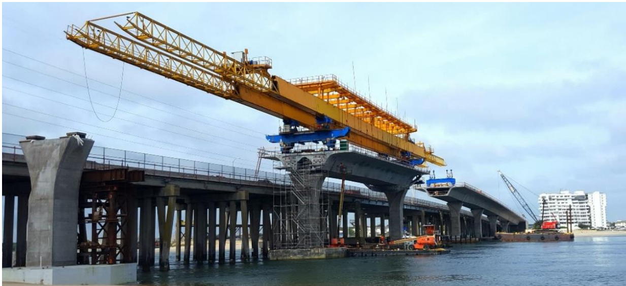
Figure 1- Lesner Bridge construction with overhead truss
