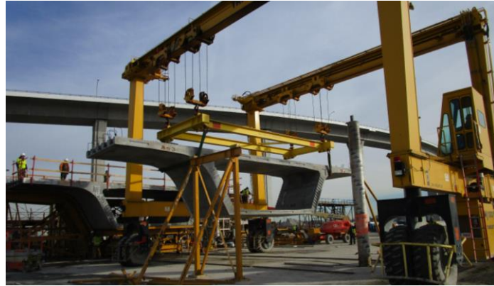
Figure 7 – Segment being lifted out of the Casting Bed
