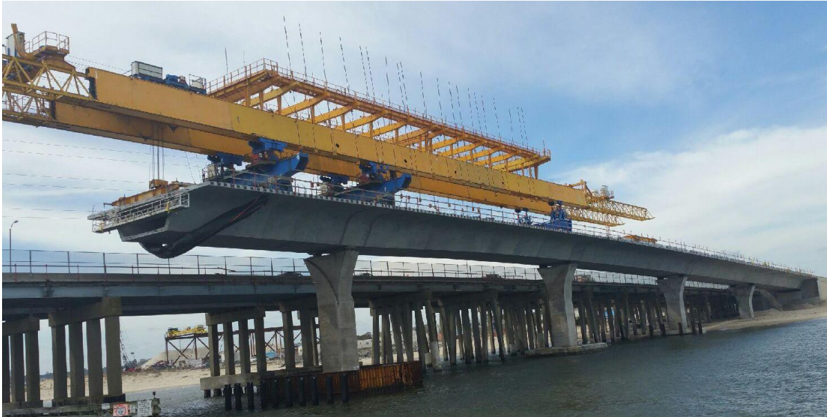
Figure 10 - Cantilever Main Span
