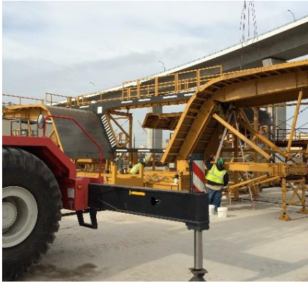
Figure 6- Segment Casting Bed
