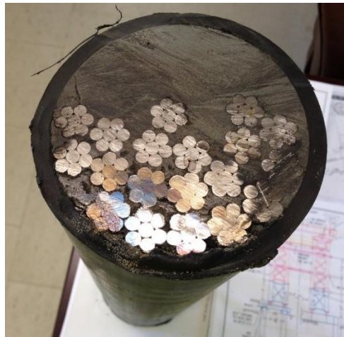
Figure 12 - Grout Tendon Cut for Investigation
