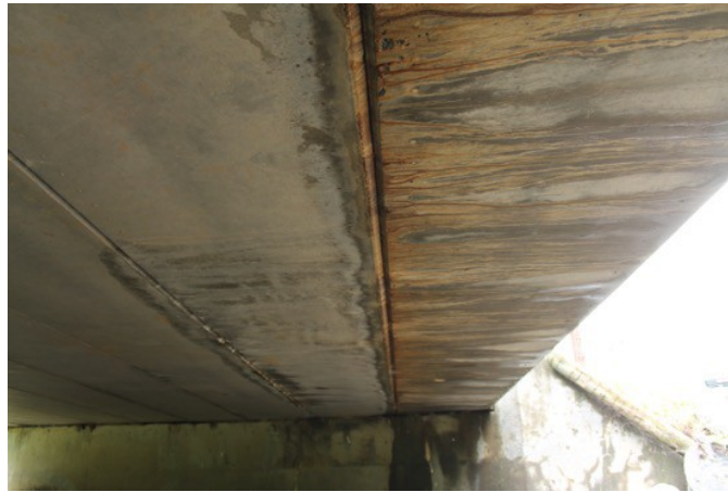
Figure 2. Leaking joint
