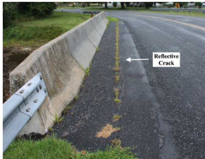
Figure 1. Reflective cracking
