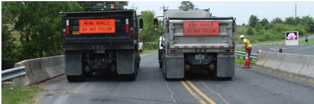
Figure 11. Test trucks crossing for Load Case 3
